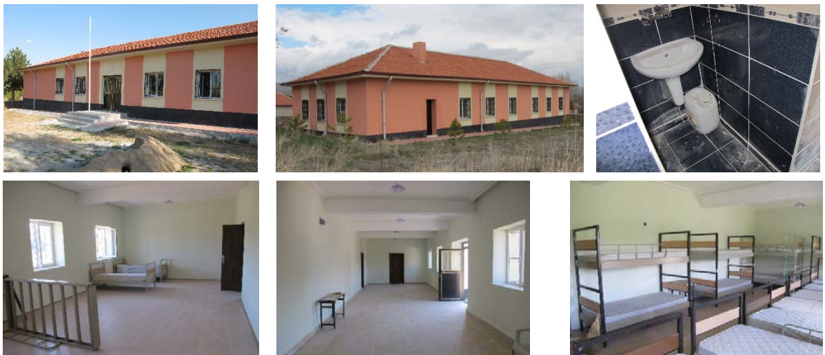
Figure 20. Şahmuratlı Village school after refurbishment (2013).
