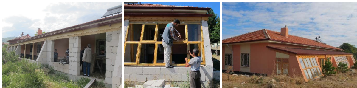
Figure 24. Construction of sunspace along south façade of former school (2014-2015).
