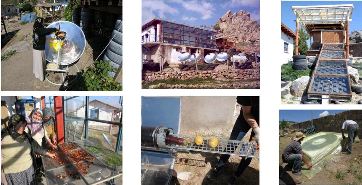
Figure 11. Solar dryers, solar cookers and hot water collectors at the Kerkenes Eco-Center.
