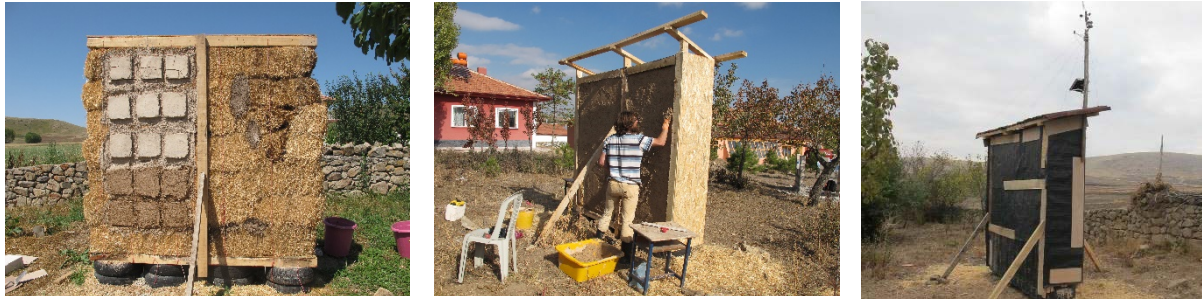
Figure 30. Research on different type of plasters suitable for straw-bale walls (2015-2016).
