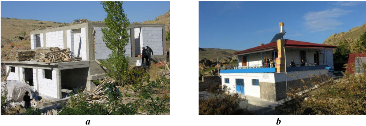
Figure 8. (a)Erdoğan Akdağ Center built with AAC blocks in 2005 and (b) completed.
