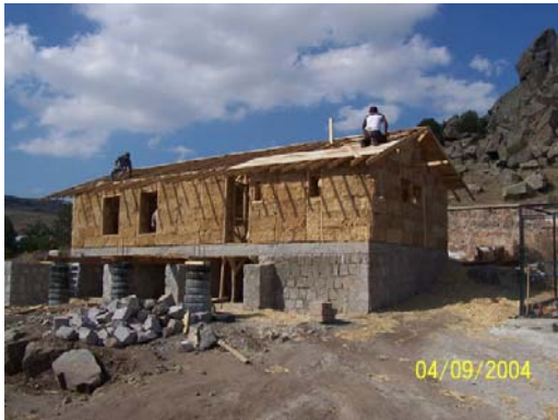
Figure 5. (a) Straw bale house built in 2004 and (b) completed in 2005.
