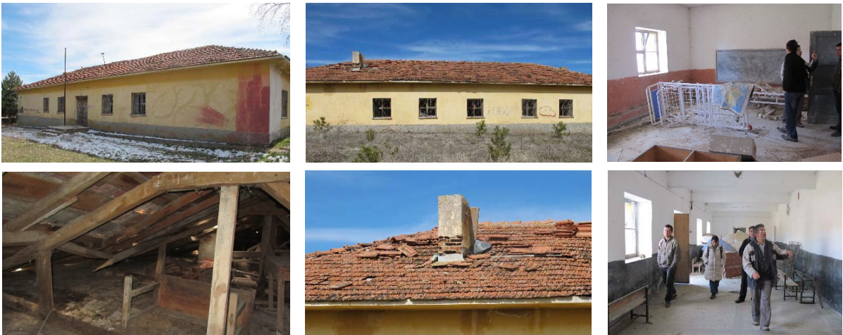
Figure 19. Şahmuratlı Village school before refurbishment (2013).
