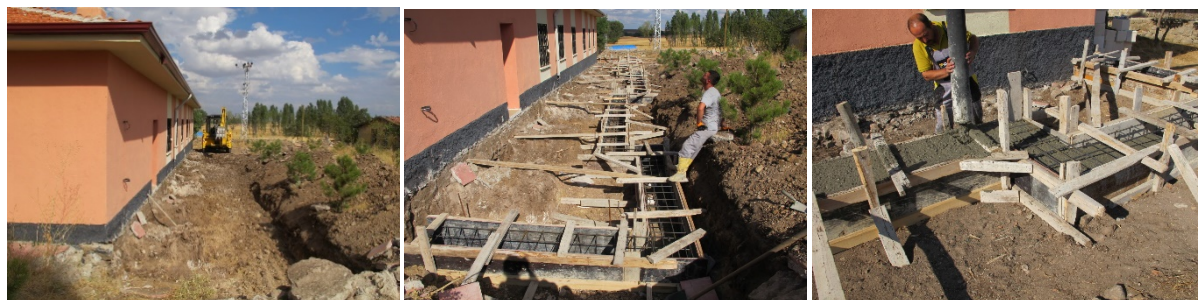
Figure 23. Vault with AAC blocks; sunspace wall; geodesic dome construction during hands on course (2014).
