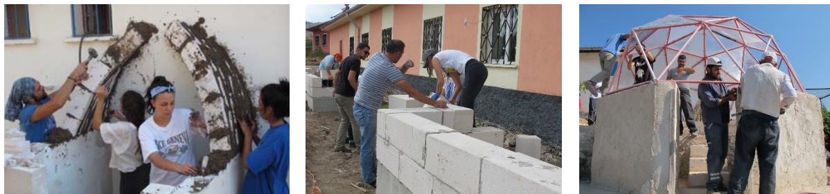
Figure 23. Vault with AAC blocks; sunspace wall; geodesic dome construction during hands on course (2014).
