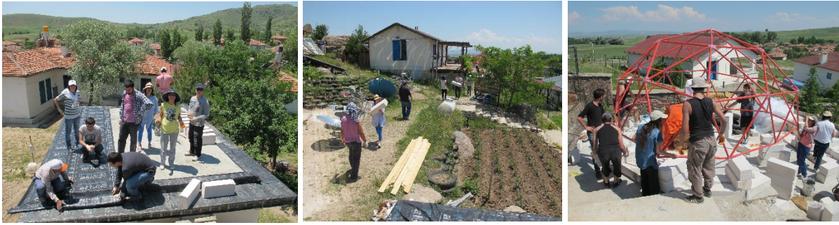
Figure 17. Repair of Eco-mud building roof and construction of geodesic dome (2012).
