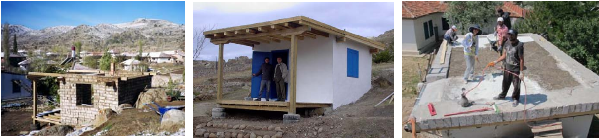
Figure 4. (a) and (b) Ecomud building built in 2002; (c) the roof was redone using AKG Gazbeton blocks during a Hands-on session with METU students in 2012.
