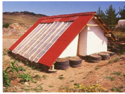
Figure 6. (a) and (b) Greenhouse built with straw bales in 2004. (c) Seedlings in the spring.
