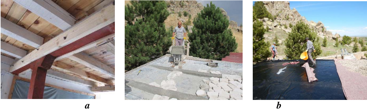
Figure 10. Solar house roof repair in 2015 and 2016.
