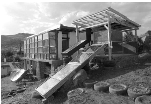
Figure 2: Surrounded by solar driers and cookers, the Kerkenes Solar Building with its south facing glazed balcony uses solar energy for heating and food processing.
