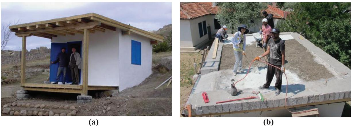
Figure 3. (a) The mudbrick building built in 2002; (b) the mud roof was replaced by AAC blocks during a Hands-on session with METU students in 2012.
