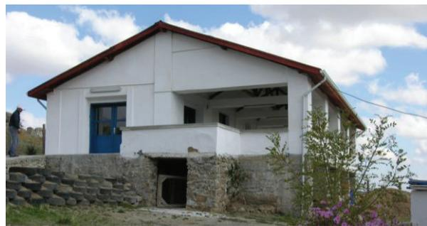
*Figure 7. A hybrid construction technique of AAC blocks and straw bales was used for the Kerkenes Stone Conservation Building.*
