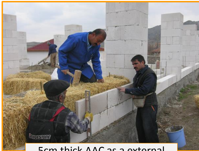
5cm thick AAC as a external facing
