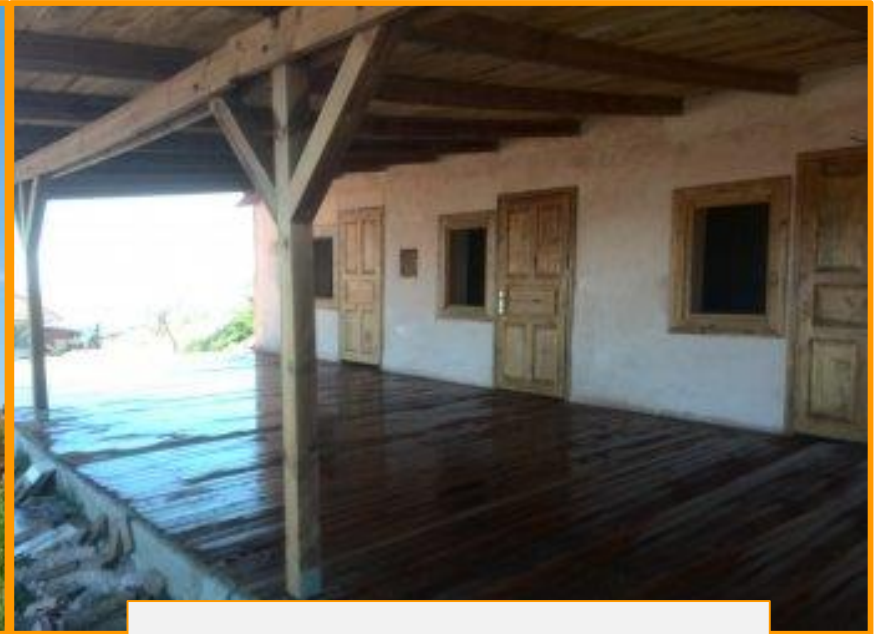
Porch on the south facing side
