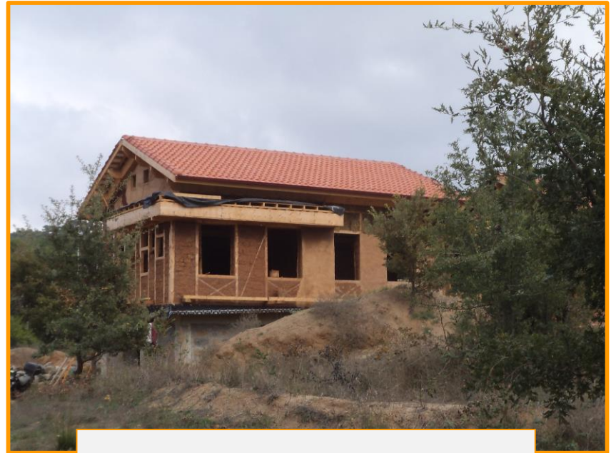
Mud-brick south wall
