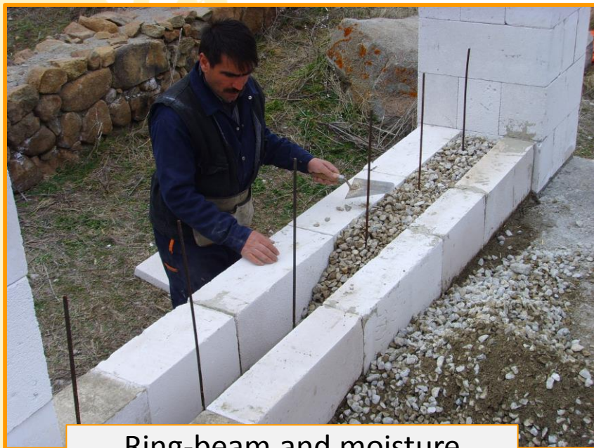
Ring-beam and moisture protection
