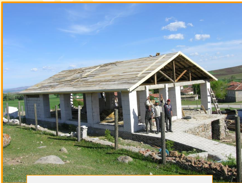
Roof build before the walls
