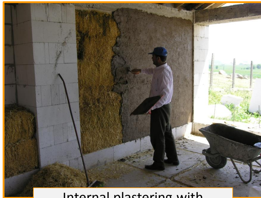
Internal plastering with cement/lime plaster
