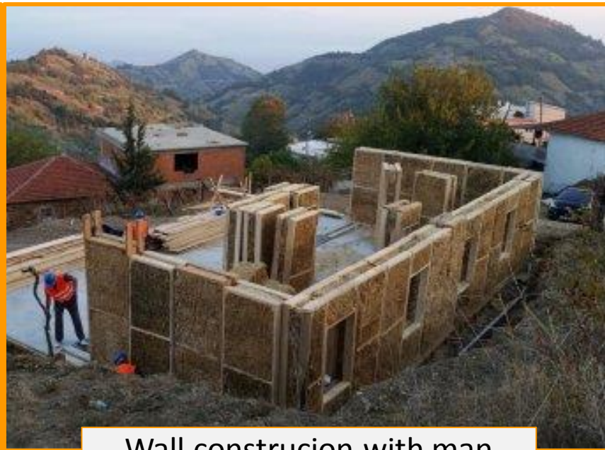
Wall construction with man power sized panels
