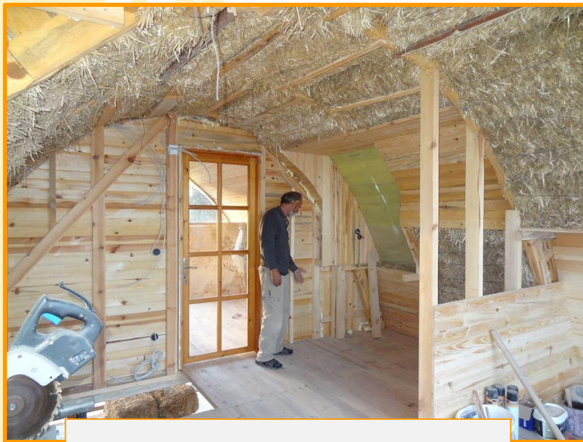
Interior wooden cladding
