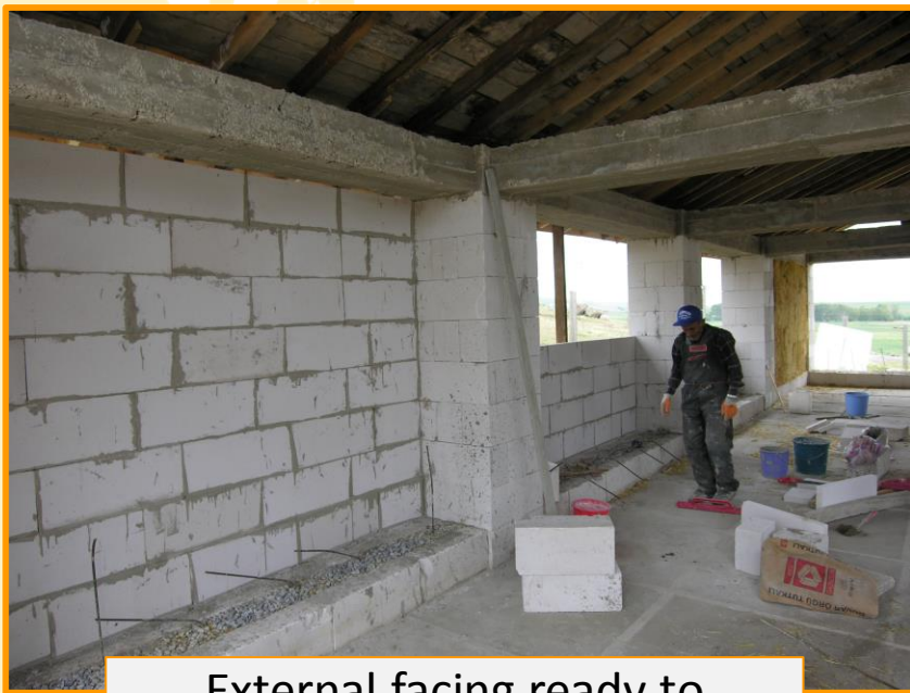
External facing ready to receive the insulation
