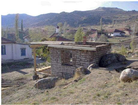
**Figure 3:** Building with mudbrick
