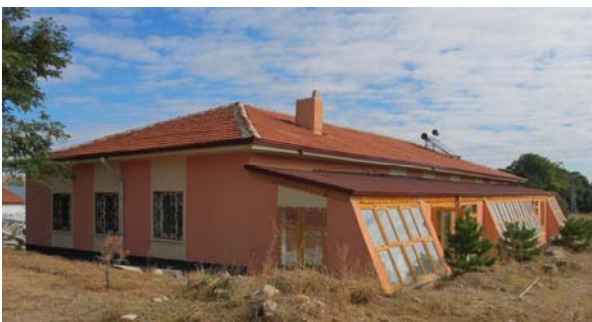
Figure 7: A solar space was added to the south façade of the school and a solar water heater was installed on the roof.
