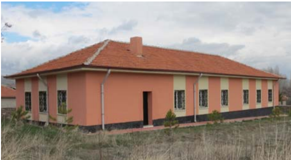
Figure 6: The village school building after renovations.
