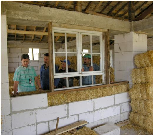
*Fig 1. A window is being installed in the under-construction hybrid wall of the Strawbale-cum-AAC building.*
