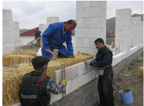
Fig 6: Innovative hybrid wall construction with AAC blocks and straw bales.
