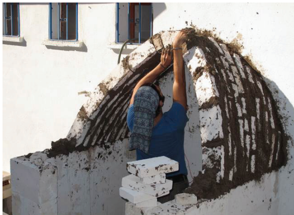
Fig 10: A Nubian vault built with AAC blocks.
