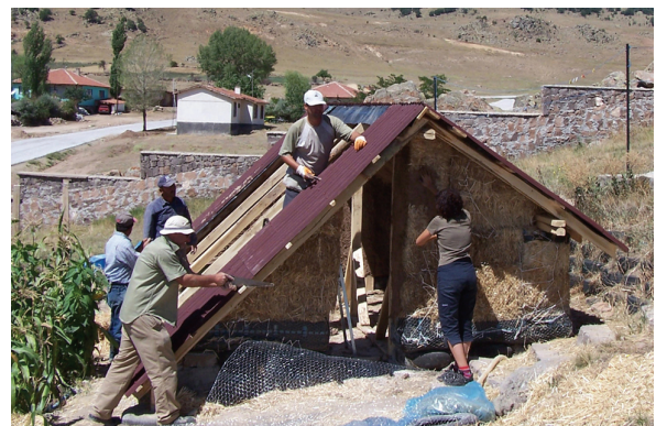
Fig 3: Construction of the Strawbale Greenhouse.
