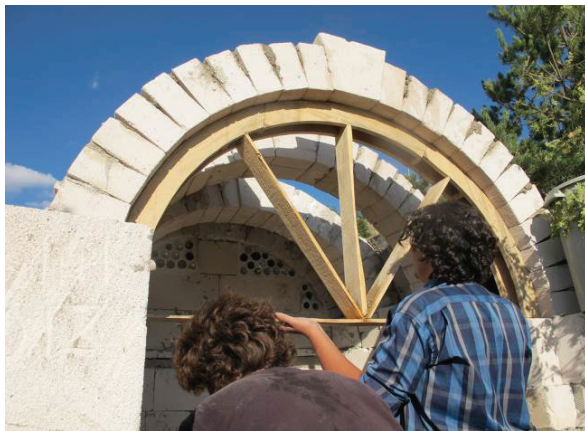
Fig 9: A vault built with AAC blocks by architecture students
