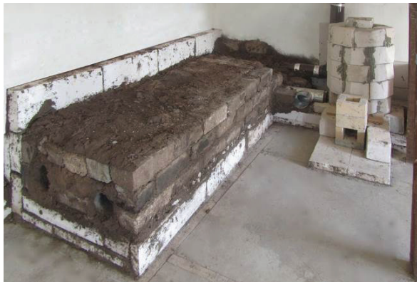
Fig 14: Rocket Stove under construction in the Strawbale House.
