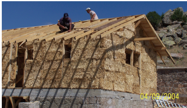
Fig 1: Construction of the straw-bale house at the Kerkenes Eco-center.
