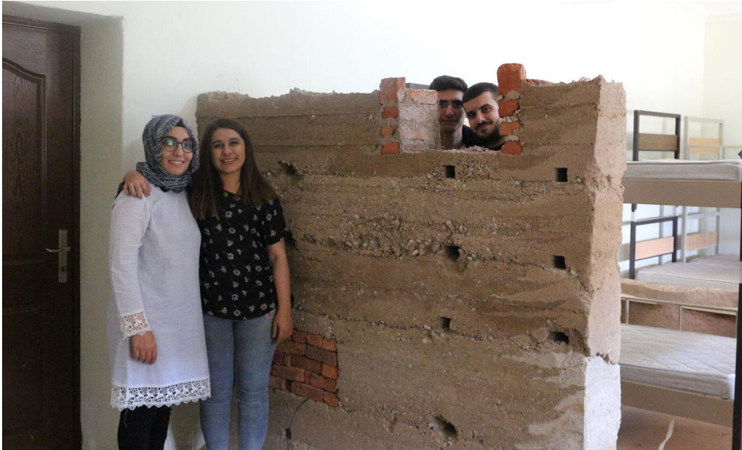
Figure 15. KTO-KÜ students heightened the existing rammed earth wall and lined the niche with bricks. (17kekc0815)
