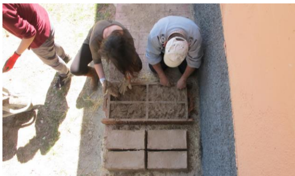
Figure 14. METU students filling mud into the mudbrick mold. (17kekc0105)
