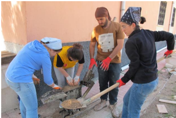
Figure 12. Soil mixture being placed into manual compressor for pressed bricks (17kekc0206)
