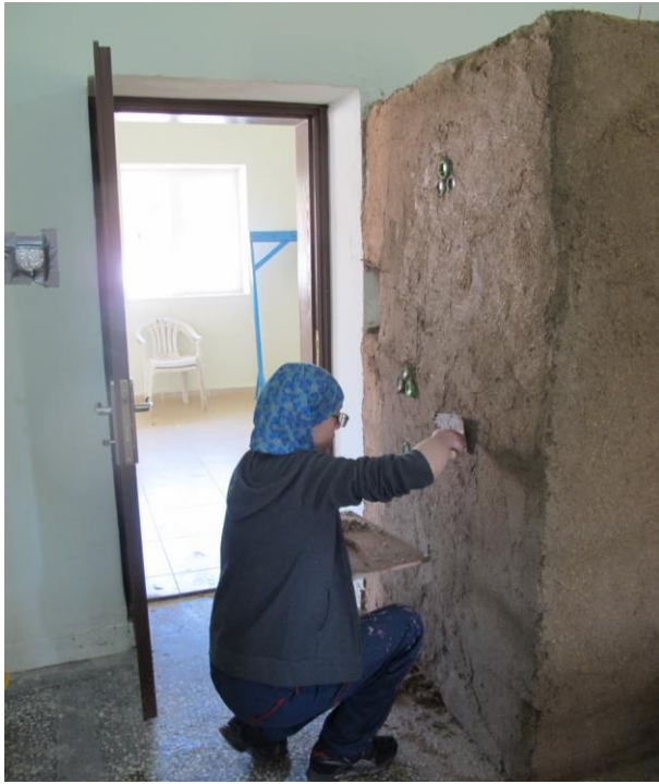
Figure 11. Mud plaster being applied on the existing slip-straw partition wall (17kekc0214)
