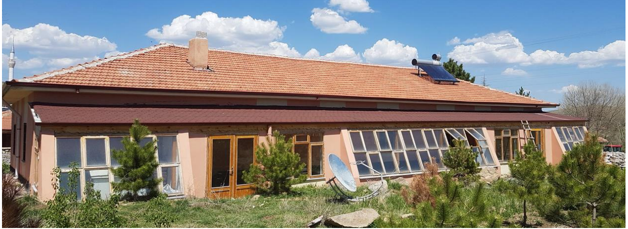
Figure 3. The rehabilitated Şahmuratlı village school, now known as the Kerkenes Training Center, hosts the Hands-on educational programs. (17kek0410)
