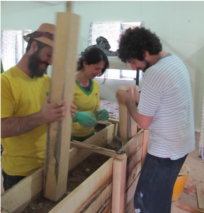
Figure 9. Students learning how to make a rammed earth wall. (17kekc0240)
