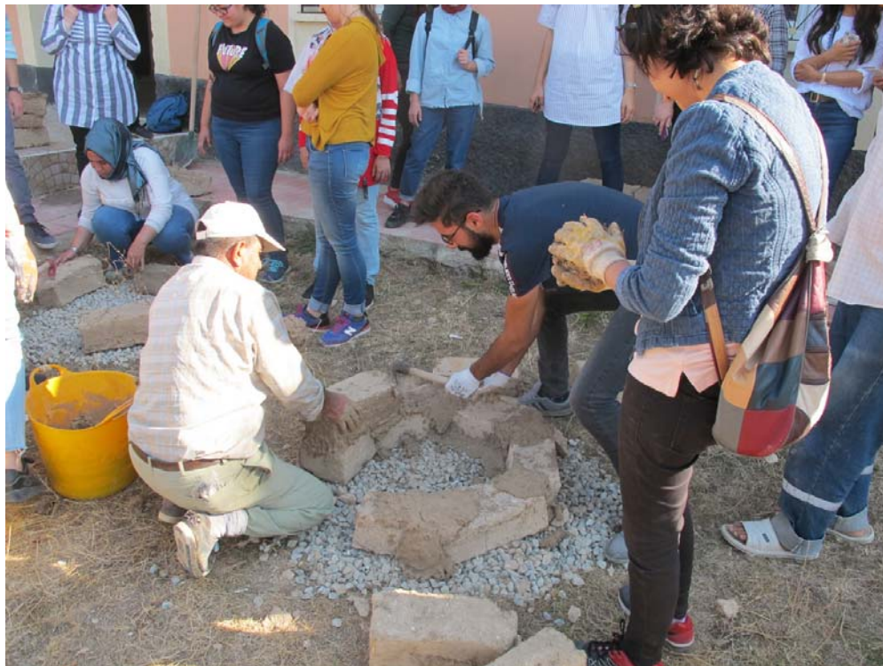
Figure 30. Making a small oven with mudbricks. (18kekc1138)
