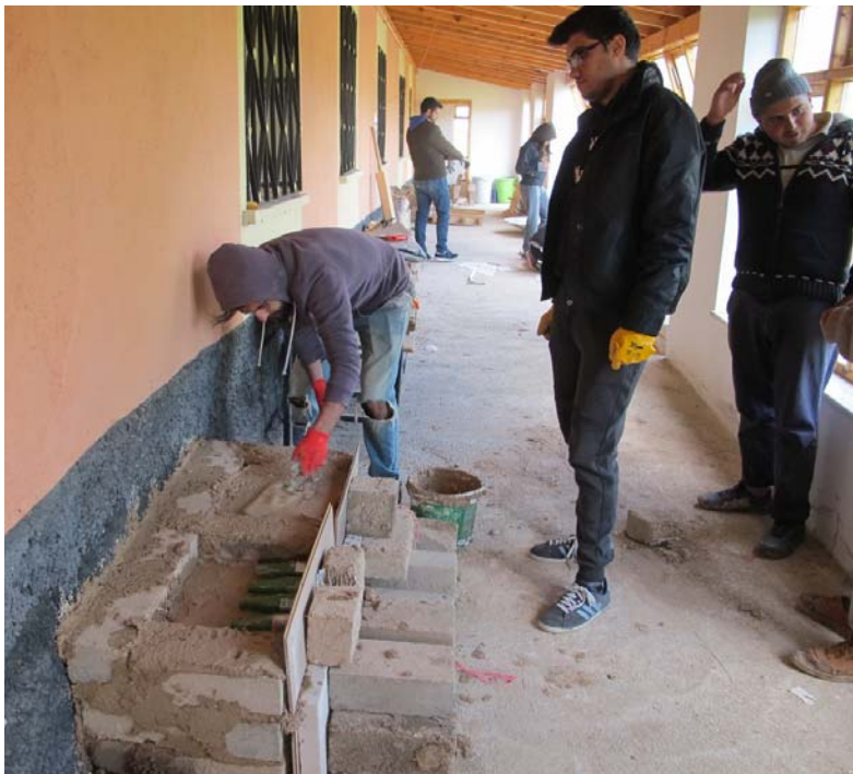
Figure 21. A bench made from mud, AAC blocks and recycled glass bottles. (18kekc0216)
