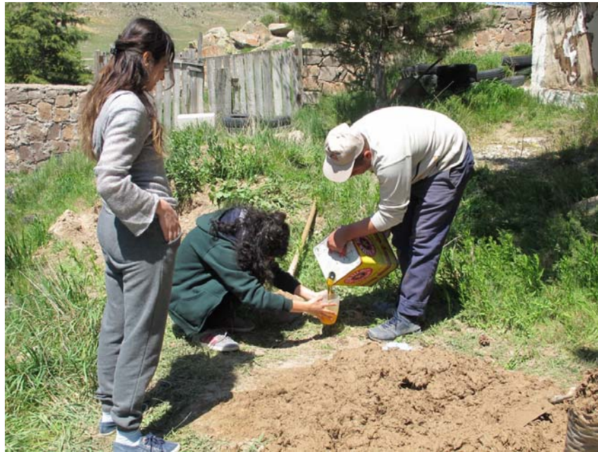
Figure 15. Mixing oil with mud plaster to increase its durability. (18kekc0241)
