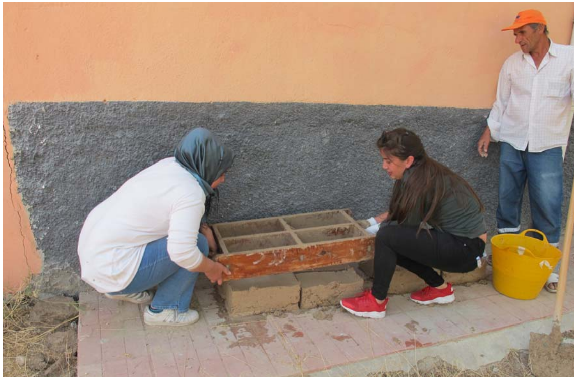
Figure 29. Making mudbricks with a wooden frame. (18kekc1133)
