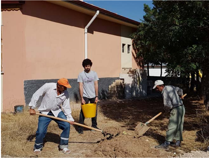
Figure 10. Villagers and the project assistant preparing mud mixtures for the students. (18kekc1003)
