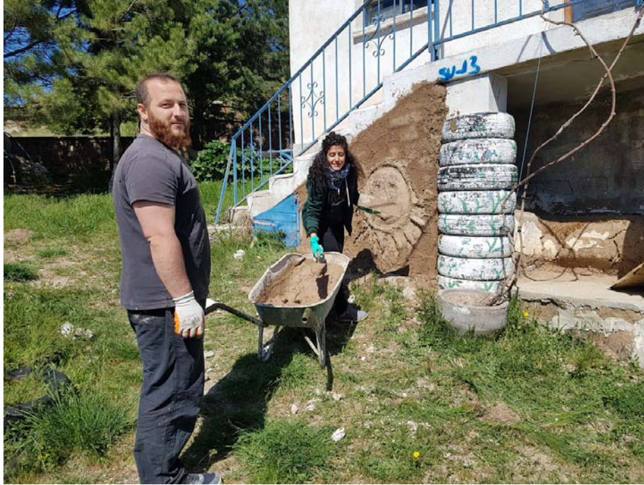
Figure 17. The mud plaster sun motif of the Kerkenes Solar House stairs was redone by some students. (18kekc0254)
