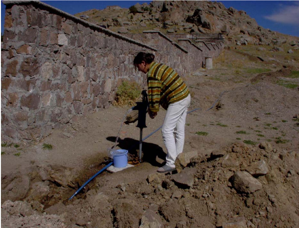
Figure 6: The first drilled hole, 7m deep, was found to produce about 2m of water and a hand pump was installed for occasional use.
