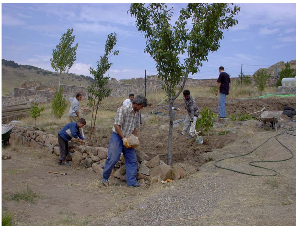
Figure 5: Terracing the Kerkenes Eco-Center kitchen garden.
