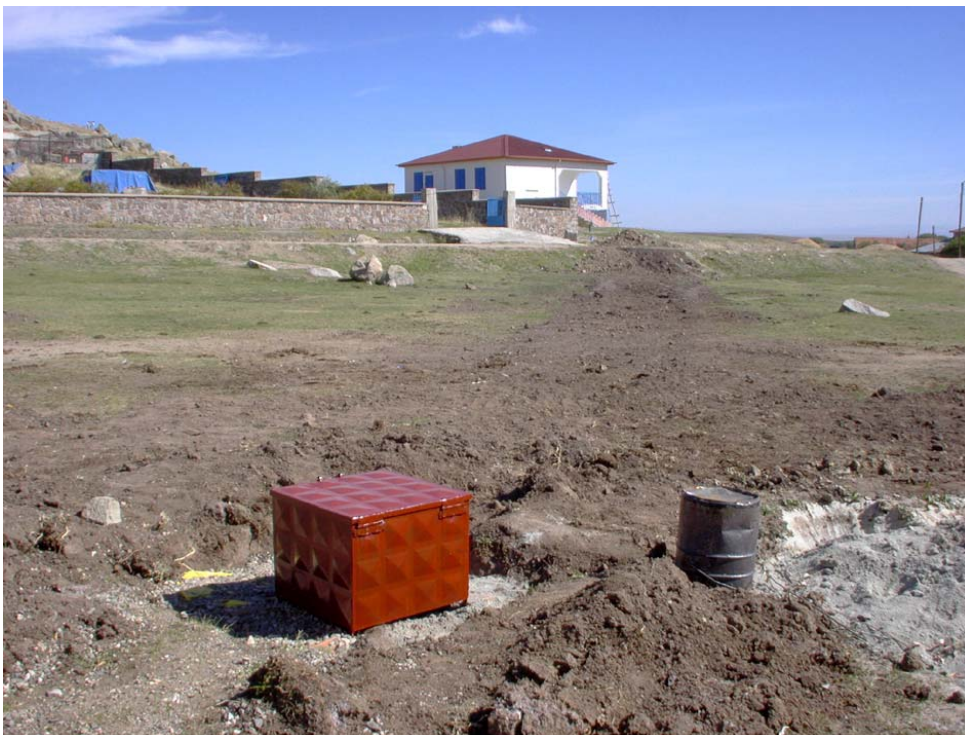
Figure 11: A buried pipe connects the pump to the existing house water tanks sitting on the hill behind the house. Water can then be gravity fed for use in the house and garden.
