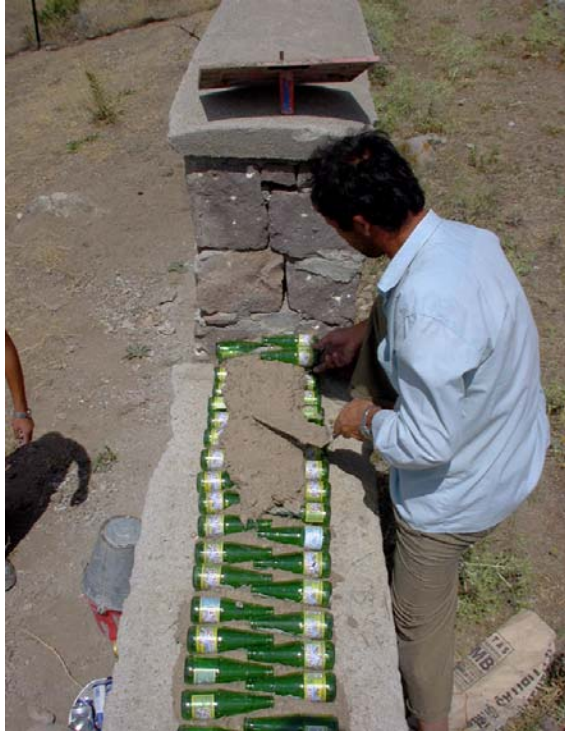
Figure 18: Building with glass bottles and mud mortar.
