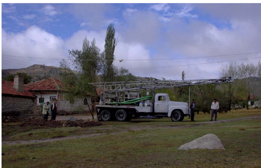
Figure 9: Job done! The drilling lorry is ready to leave.
