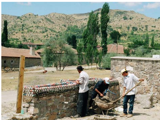
Figure 10. Bottles and cans from drinks consumed during the summer season of archaeological fieldwork are recycled in the garden walls enclosing the expedition house compound.
