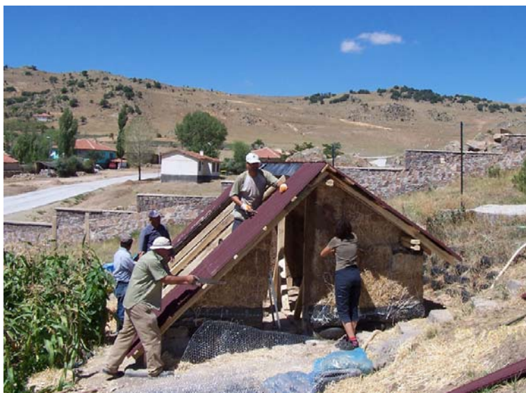
Figure 27. Workers from the Şahmuratlı village, students from METU and other participants learnt as much as possible from Bora Topluoğlu as they worked together to build the small strawbale greenhouse in August 2004.
