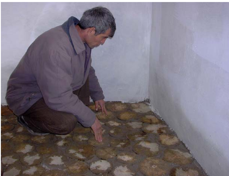
Figure 15. The floor consists of the timber blocks embedded in a mixture of mud and lime. (03kejv0601)
