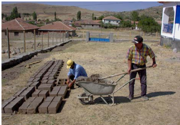
Figure 9. Mudbrick made during the 2002 and 2003 summer seasons were used to build the Eco-Building completed in the autumn of 2003. (03jv0310)
