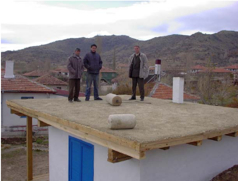
Figure 13. The building has traditional mudbrick walls and a mud roof which has to be regularly rolled to ensure that it does not leak. (03kejv0609)
