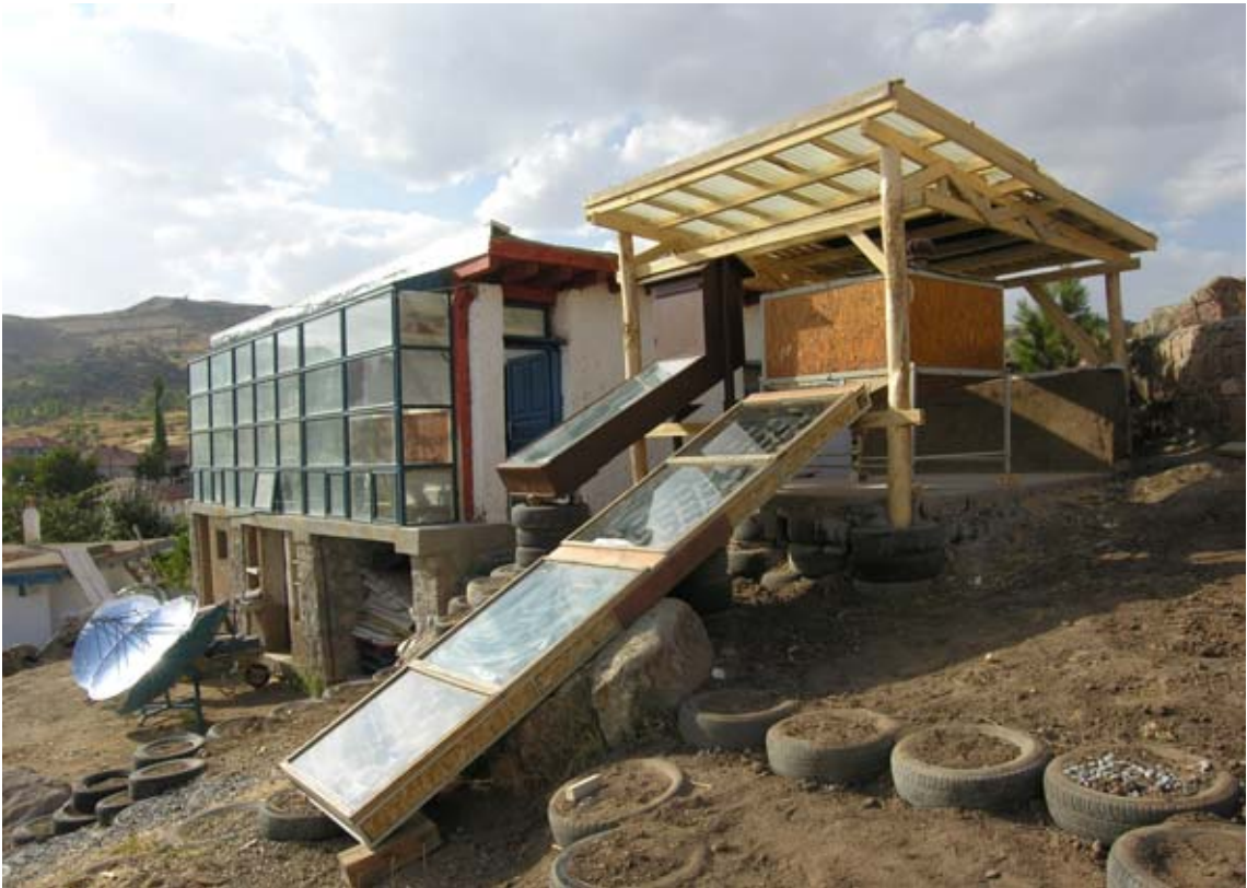
Figure 8. Solar Building, solar driers and solar cookers at the Kerkenes Eco-Center. (08kenc1808)
