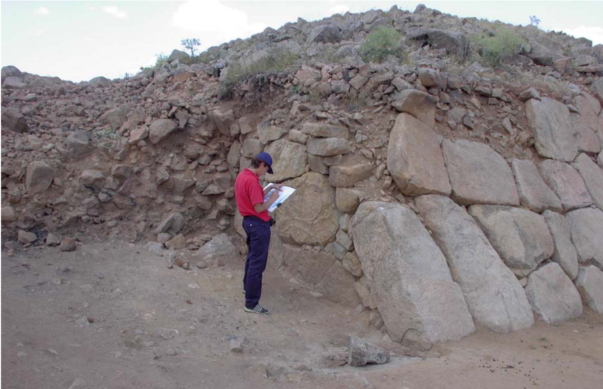
Figure 46: Gülnur Uçar drawing the glacis over a rectified photograph before consolidation. (02dpjv2519)
