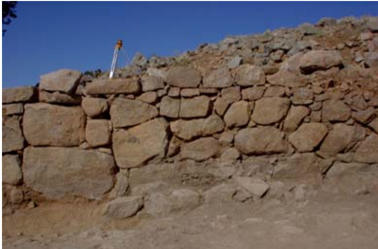
Figure 6. The north-west wall of the gate passage where, at left, the gully has eroded down below the base of the wall which, at centre, has been protected by the addition of a row of stones. The vertical junction in the wall face at the extreme left is where the glacis butts against the front of the tower wall. (03dpjv6303)
