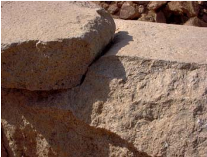
Figure 56. The top of a granite orthostat carefully cut to seat a thinner levelling course. The face of each stone has broken away as a result of the intense burning. (03dpjv5123)
