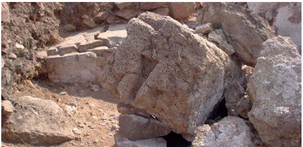
Figure 19. A fallen block of conglomerate has two clamp cuttings, that on the top left being incomplete. The granite block seen in Fig. 18 is in situ in the tower wall behind. (04dpjv2215)
