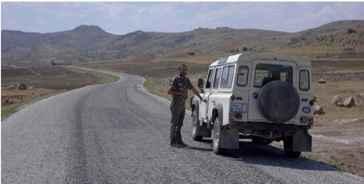
Figure 5. The new tarmac road winds all the way up to the site, allowing a comfortable ride for cars and coaches driving up to the city wall at the base of the Kale, the prominent hump on the horizon. (04dpjv3304)
