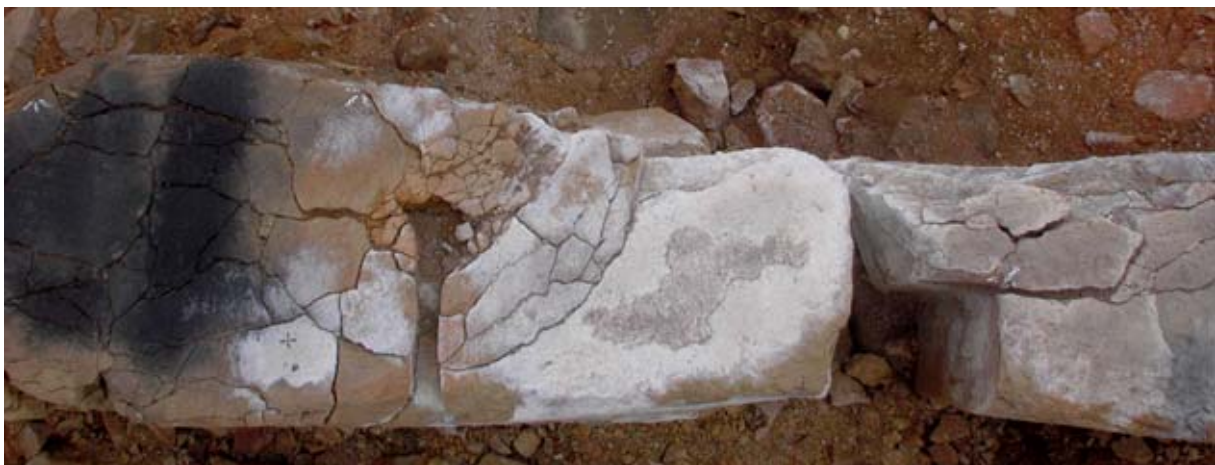
Figure 17. A square cutting was carved out of one of the sandstone blocks of the South Tower wall presumably to locate either a vertical timber or a floor beam. To the left, a clamp cutting perhaps held a wooden clamp that tied the block to floor joists. The soft sandstone has been shattered by the fire and is encrusted with salts. (04dpjv2848)
