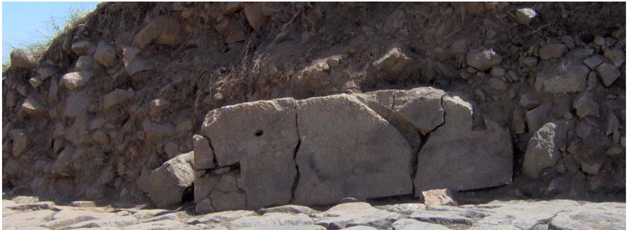
Figure 43. Clamp cuttings on a block fallen from the South Tower. (05dphp2111)
