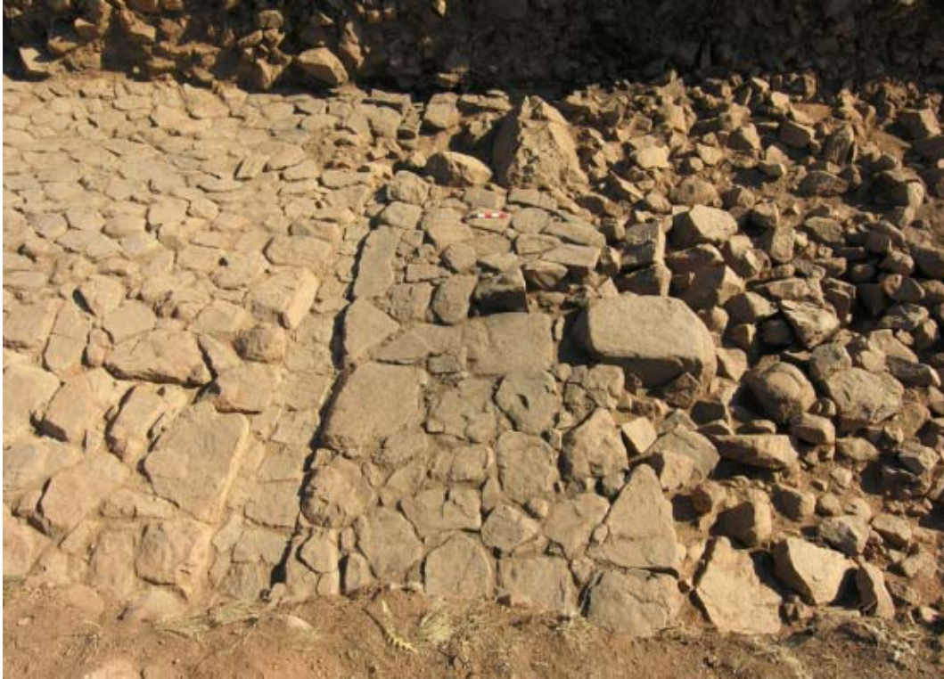
Figure 38. A drain set into the pavement along the rear façade took surface runoff away from the entrance in a northerly direction. (05dpnc0218)
