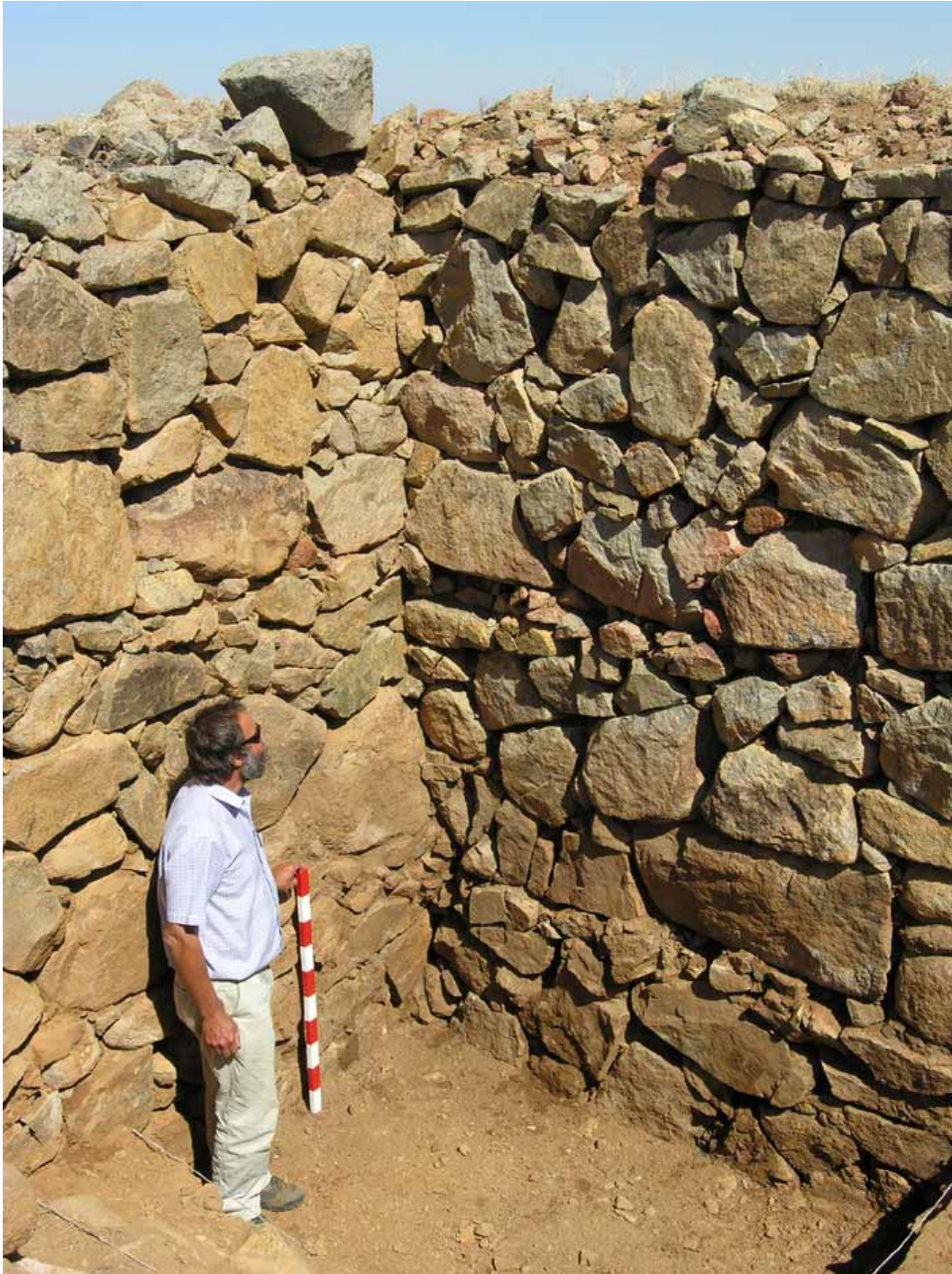
Figure 40. New stretches of wall faces at the inner chamber of the Cappadocia Gate were exposed in TR13. (07dpnc0660)
