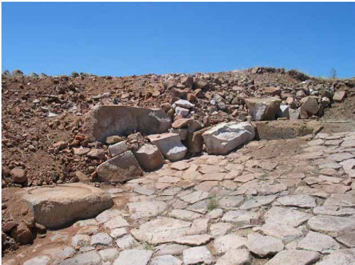
Figure 37. In the Monumental Entrance fire-shattered blocks were moved to the sides while the rubble core of the platforms was ramped to increase safety. (07dpnc1748)
