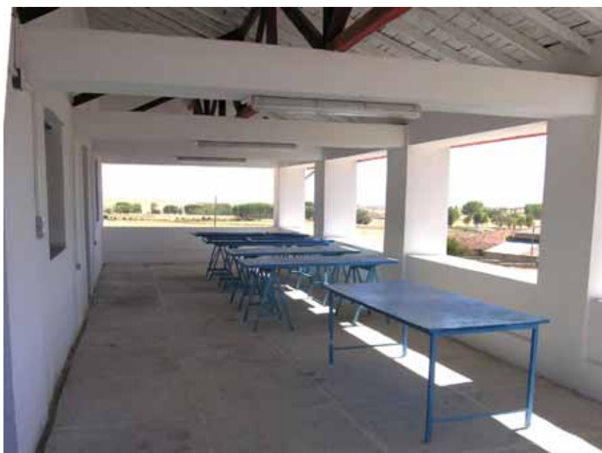
Figure 16. As well as the large spacious workshop, the building provides an equally spacious covered balcony where tables can be laid out for sorting and mending architectural stone elements. (07dpnc1031)
