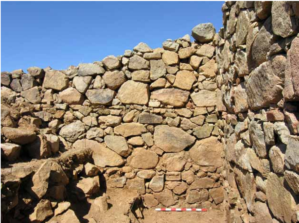
Figure 41. North East wall face of the inner gate chamber in Trench TR13. Courses of smaller stones could indicate the location of horizontal timbers. (07dpnc0656)
