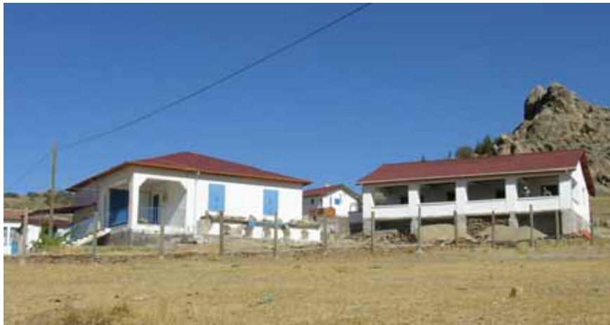
Figure 14. The new Conservation Workshop, at right, is adjacent to the Kerkenes Conservation Laboratory and Depot building, at left. (07dpnc1023)
