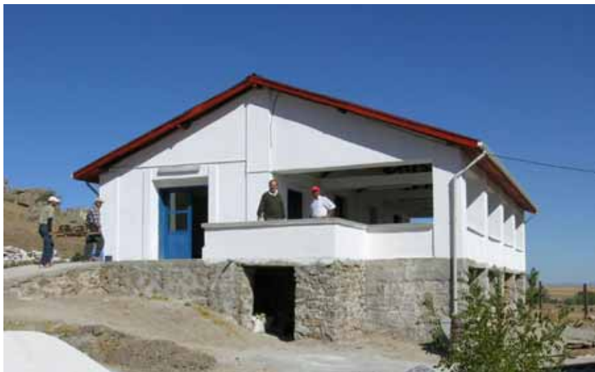
Figure 15. Doors and windows were finally put in place and painted in the autumn, before the first snow. (07dpnc3206)
