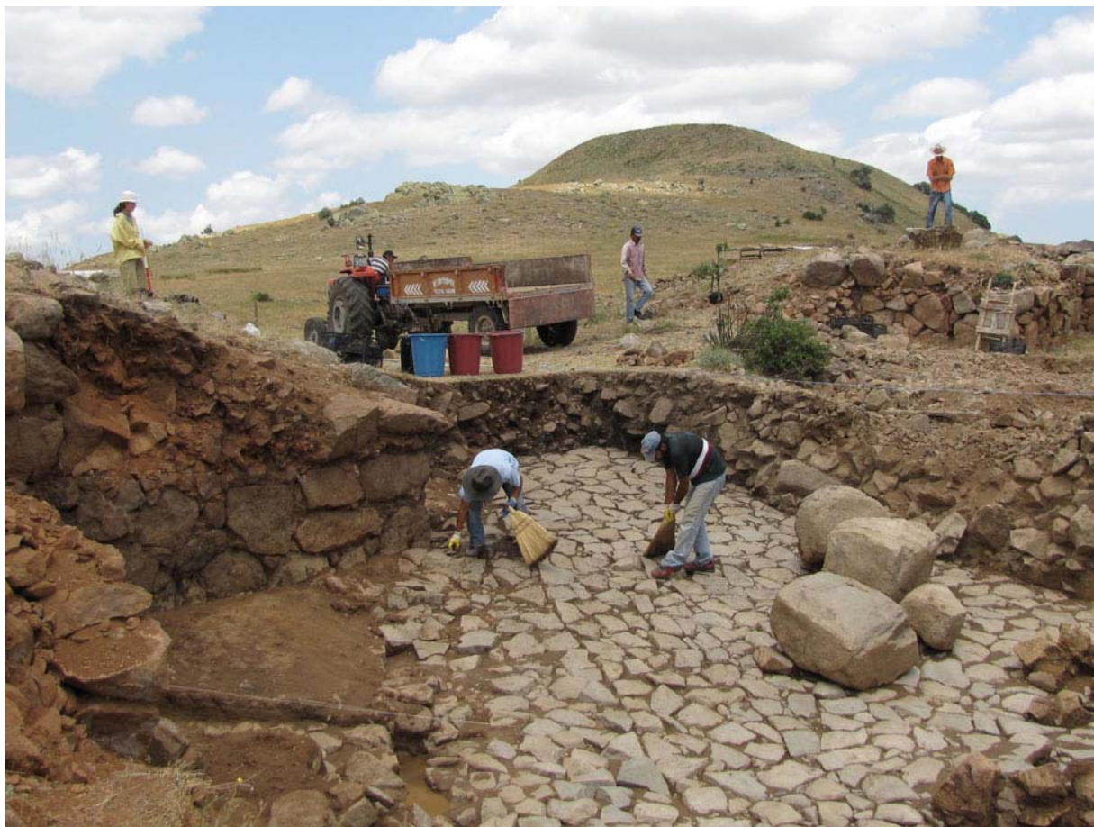
Figure 39. Cleaning the paved gate passage and partially capped drain. To the left a section through the clean light clayey material that lay over the pavement was recorded before further cleaning was undertaken. (09dpcp0633)
