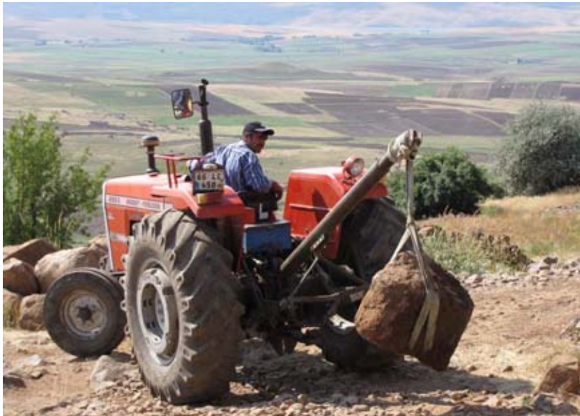
Figure 28. Stacking large fallen stones for later use in repairs. (09dpcp0233)
