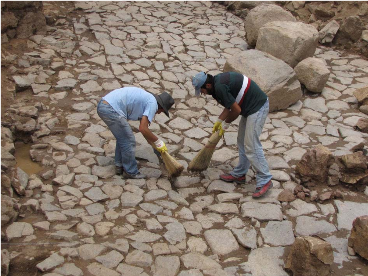
Figure 24. Paving stones uncovered in the gate passage are angular and of moderate size. (09dpcp0642)
