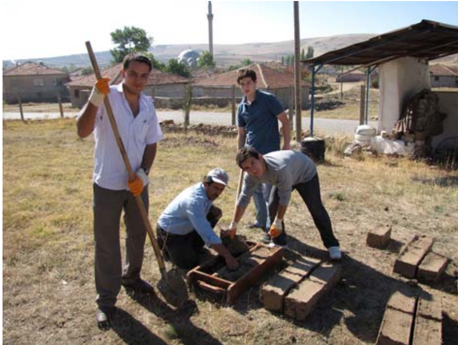
Figure 6. Architecture students from METU learning how to make traditional sun- dried mudbricks. (09kecp0714)
