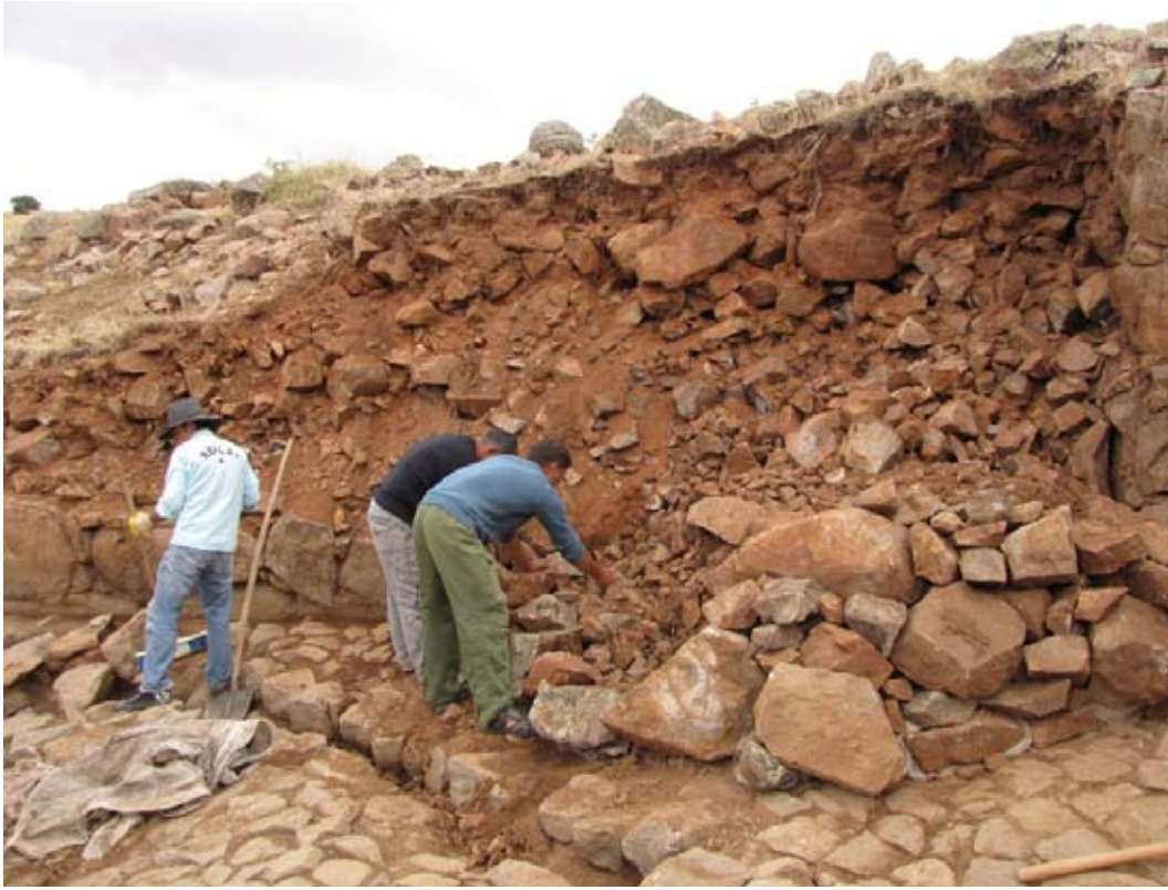
Figure 30. The very loose stone core of the southwest wall was exposed when the facing, in which horizontal timbers were incorporated, had collapsed. (09dpcp1619)
