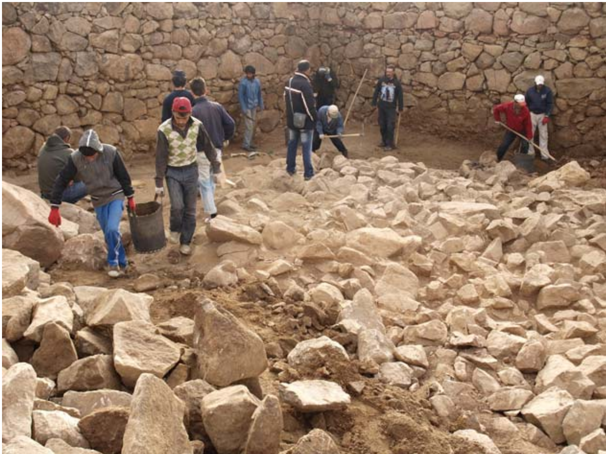
Figure 94. Cleaning the last of the fallen stone in the Gate Court. (10dpkc2227)
