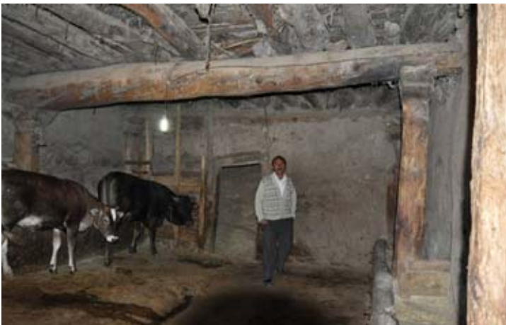
Figure 66. Kara Mehmet in his stable, now used as a cowshed, at Şahmuratlı village. A central drain runs the length of the concrete floor while food troughs run down either side. The doorway at the far end leads into a dry store for fodder. Note the size of the juniper roof beams which are no longer available in the immediate region today. (10dpnd1904)
