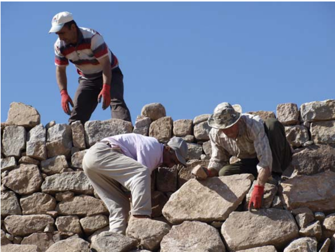
Figure 149. Where the sloping glacis joined the vertical wall stones were carefully selected to fit in the gap. (10dpkc1936)
