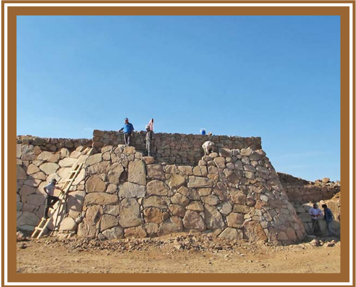
Figure 1. Restoration of the Cappadocia Gate glacis in progress. (10dpcg0425)
