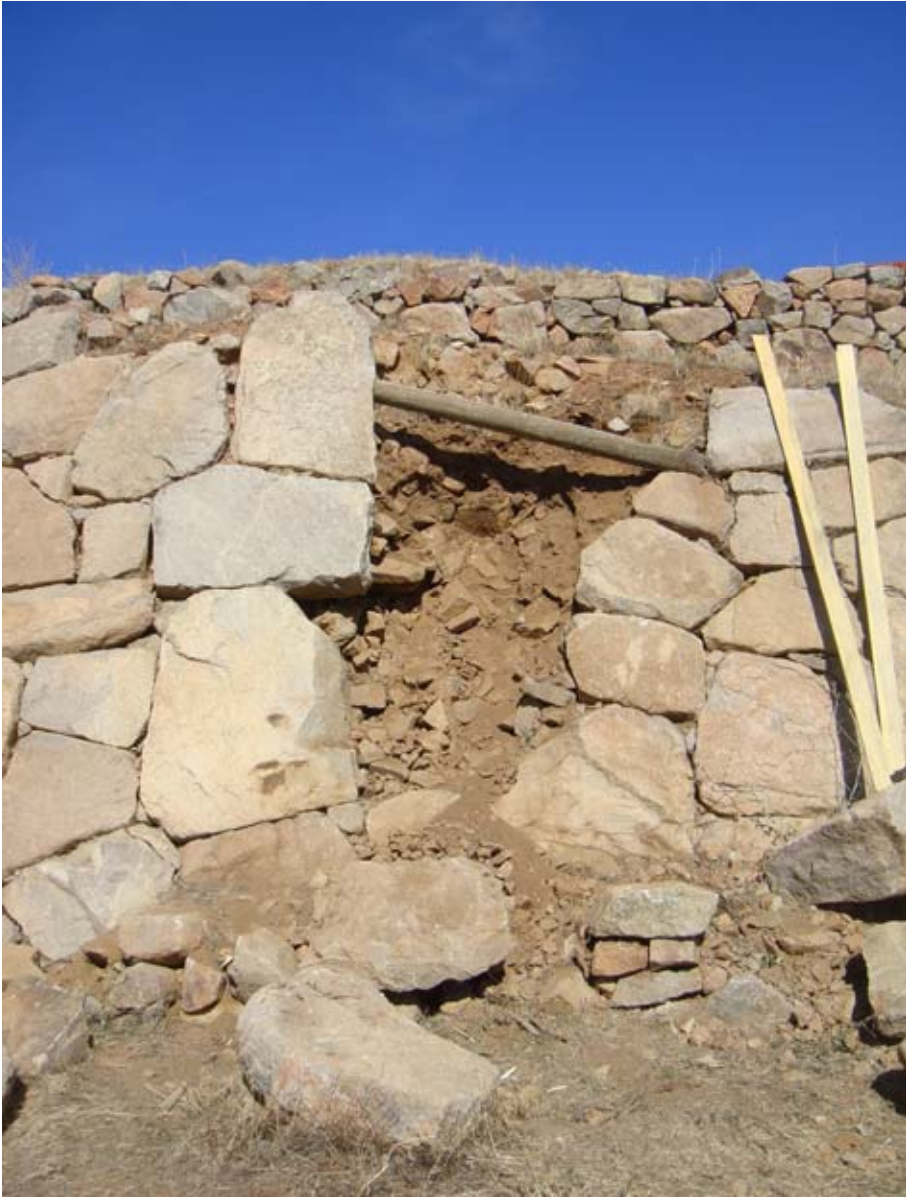
Figure 141. The large stones that had slipped down from the southeast face were identified from photographs taken in 1999 and put back in place. (10dpkc3513)
