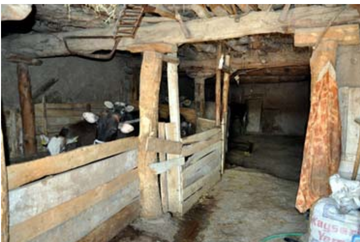
Figure 68. Detail of temporary wooden partitions, here used to separate calves from their mothers. (10dpnd1915)
