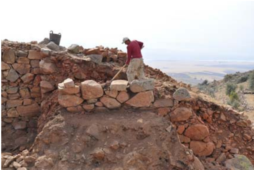
Figure 98. Once fully recorded, the upper courses of stones from the northeastern wall of the Middle Tower were moved back before the remaining fill was removed. (10dpnd1245)
