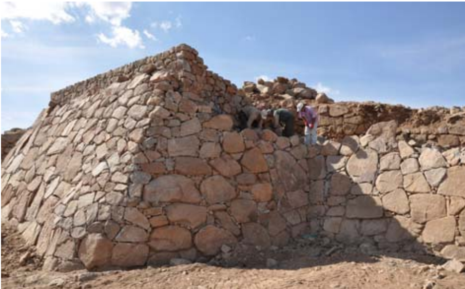
Figure 153. The glacis was rebuilt to its full height across the junction between the East Tower and the City Wall. (10dpnd1422)
