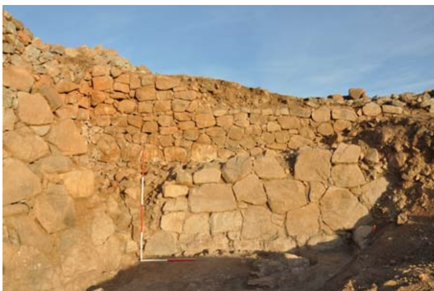
Figure 115. The junction of the East Tower and adjacent stretch of the City Wall after excavation revealed the surviving portion of the glacis. (10dpnd1012)
