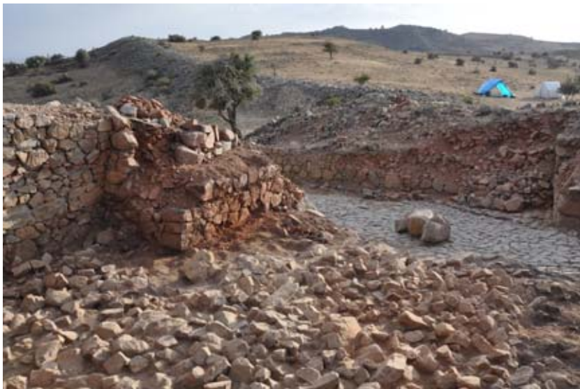
Figure 96. The base of the collapse in the Gate Court with a portion of the paving revealed in 2009. The locations of sandstone blocks fallen from the Middle Tower were carefully recorded. (10dpnd1388)
