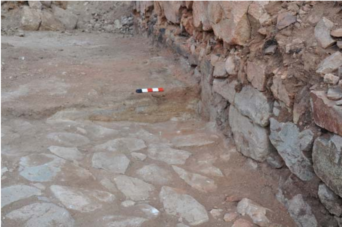
Figure 109. Silty clay derived from mud plaster on the pavement in front of the Middle Tower. Traces of mud plaster cling to the wall face while reddish destruction debris fill a depression caused by large falling stone (removed). (10dpnd2012)
