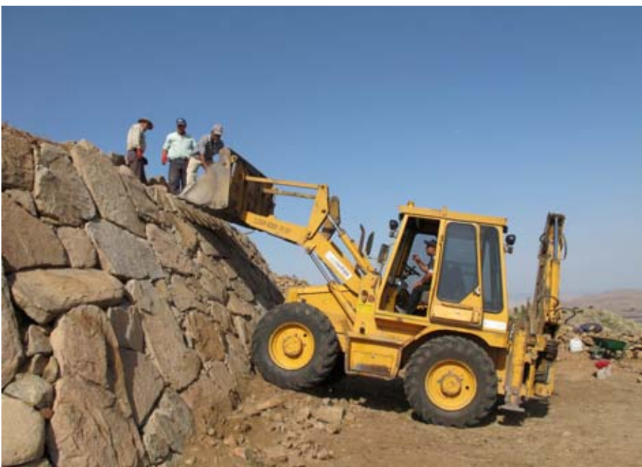
Figure 142. The machine's bucket was an efficient substitute for scaffolding. (10dpcg0328)
