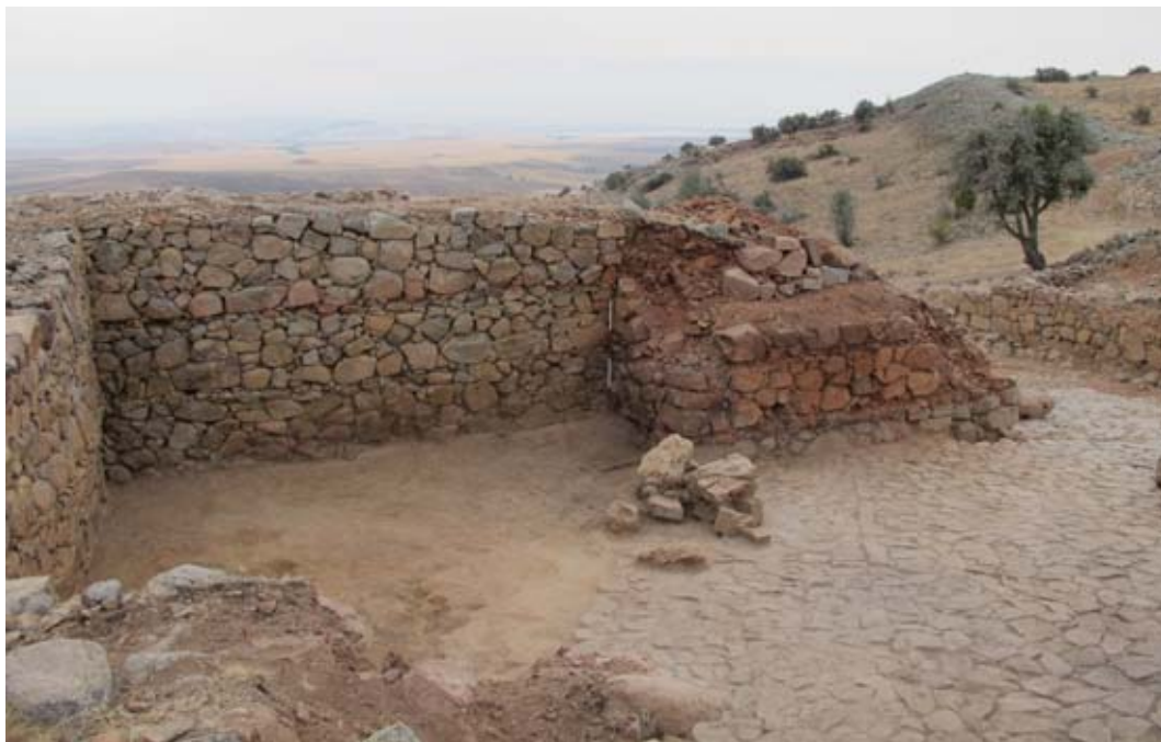
Figure 125. Looking towards the Middle Tower from which sandstone blocks, at centre, had fallen. Note the line of the paved road and the curved edge of the eastern extension. (10dpcg0729)
