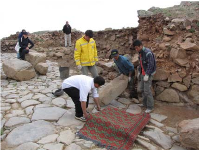
Figure 158. The aniconic stele was removed from the Cappadocia Gate passage after it became dislodged when the corner of the Middle Tower collapsed. (10dpcp0812)
