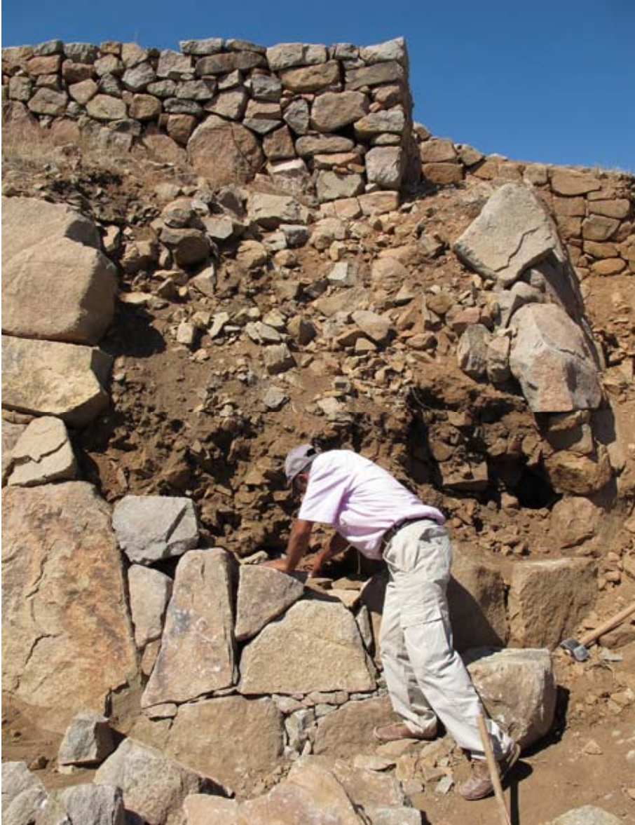
Figure 139. Restoration of the glacis was essential if the very loose fill of rubble and soil was to be stopped from washing down. (10dpcg0301)
