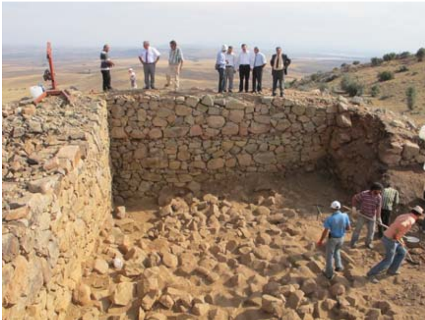
Figure 95. The base of the collapse from an elevated vantage point. At centre right the corner of the Middle Tower from which sandstone blocks fell on the surface during the destruction. (10dpcg0357)
