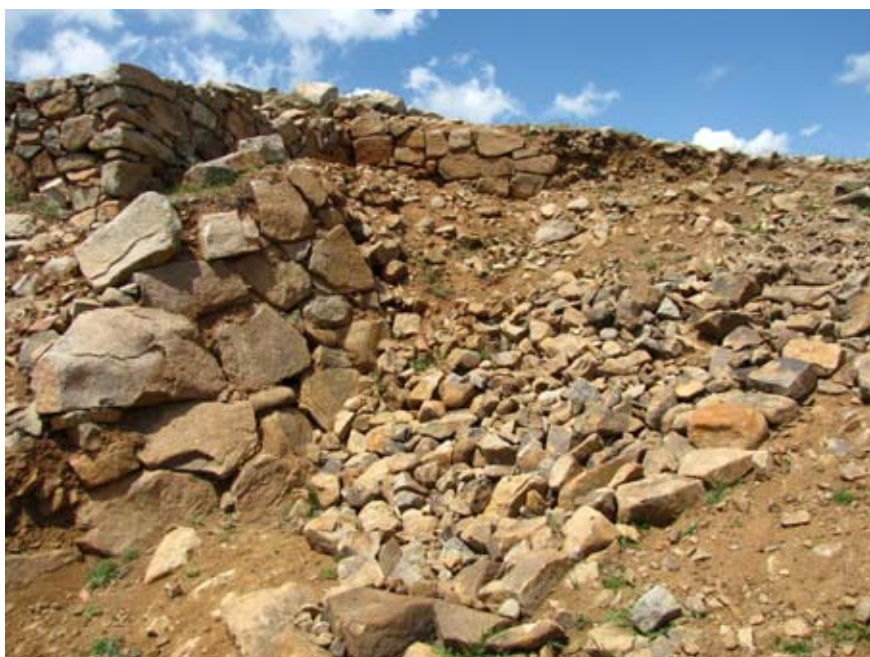
Figure 114. The east corner of the East Tower photographed in May 2010, before excavation of the glacis. (10dpcp0304)
