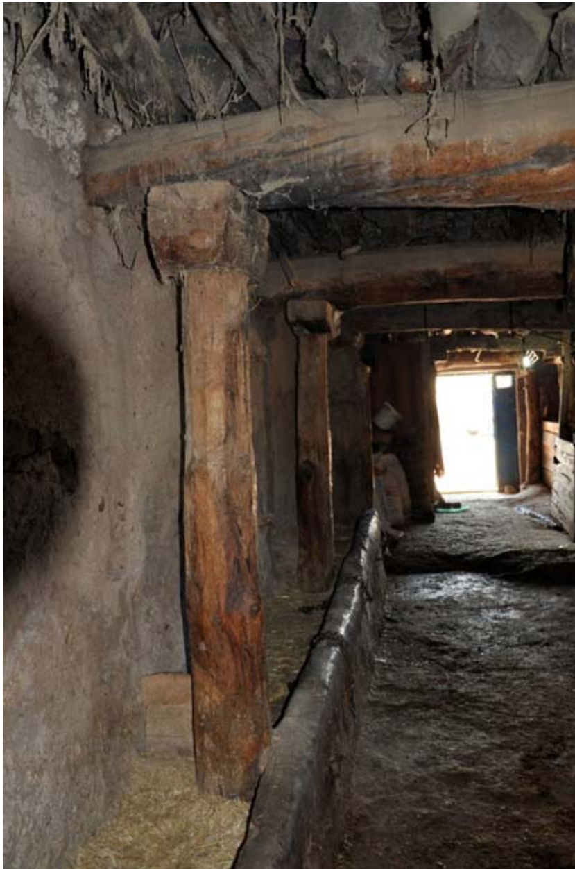
Figure 64. Detail of wooden pillars, capital and roof beams with mud-plastered wall and food troughs. (10dpnd1907)
