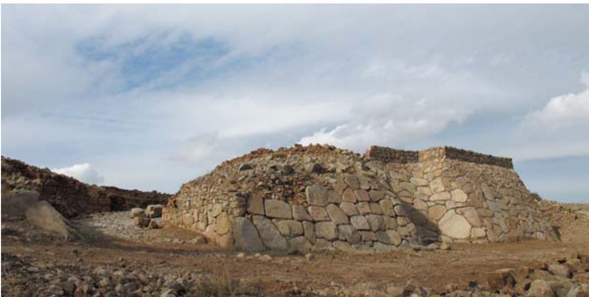
Figure 127. The Cappadocia Gate glacis photographed in October when the 2010 restoration work was completed. (10dpcg0933)
