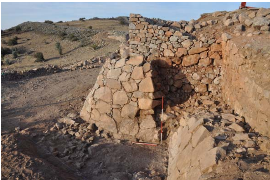
Figure 117. Excavation at the junction of the East Tower and the City Wall revealed a working transverse face in the tower glacis. (10dpnd1029)
