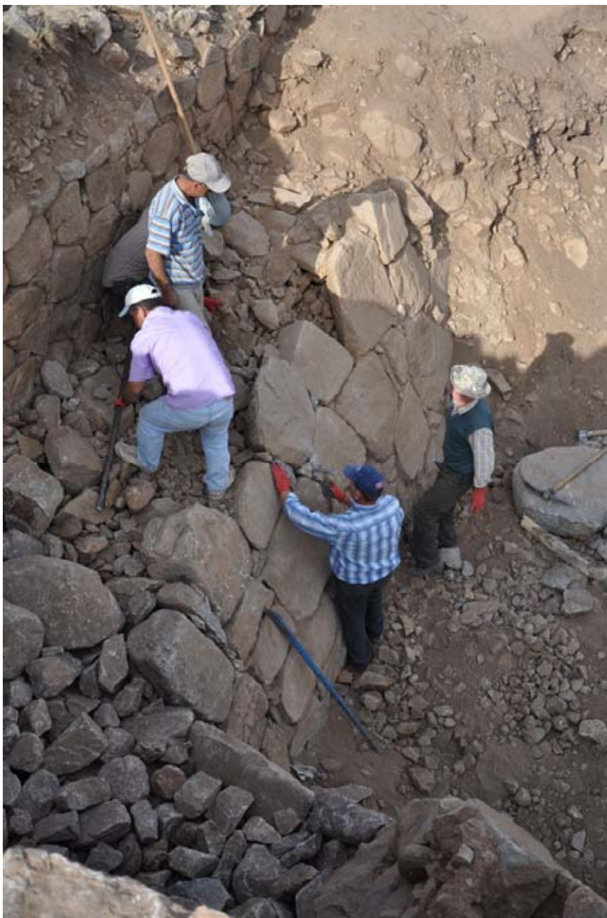
Figure 151. The masons filled in the space behind the large glacis stones with medium and small stones. (10dpnd1376)
