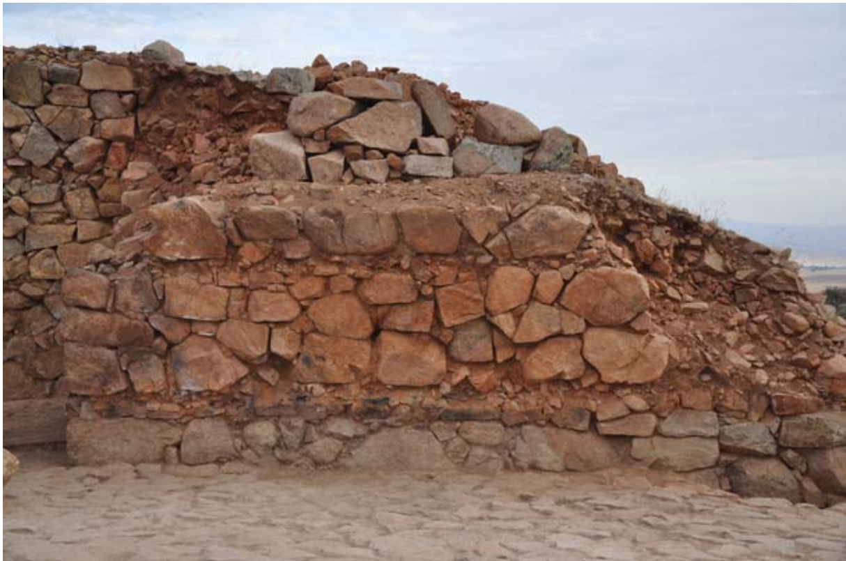
Figure 106. The inner face of the Middle Tower before it collapsed showing horizontal beam positions and the intensity of the fire. (10dpnd2168)
