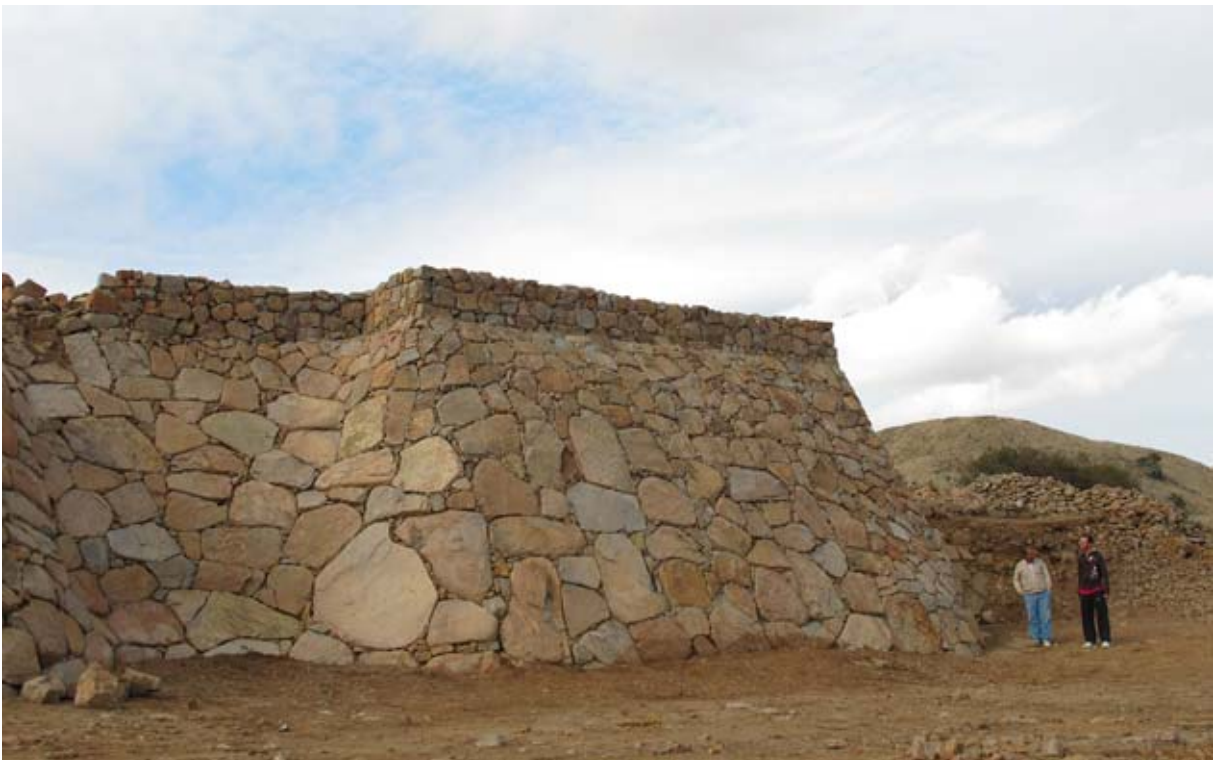
Figure 156. The Cappadocia Gate glacis restored to its original height. (10dpcg0938)
