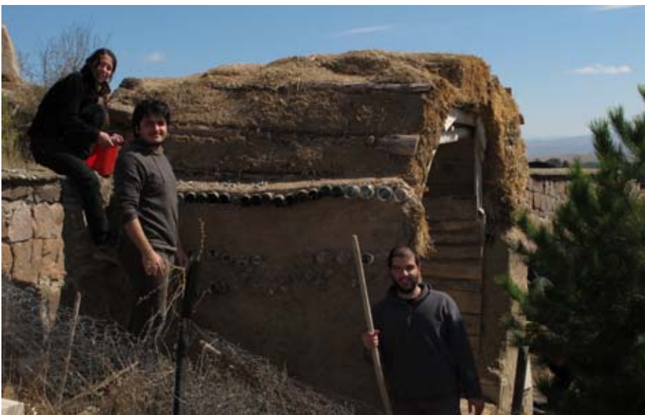
Figure 13. Working in groups, students build with straw bales, mud, and recycled bottles and cans. (10kecg0622)
