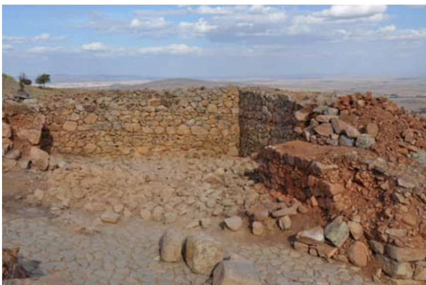
Figure 97. The base of the collapse looking east. (10dpnd1434)
