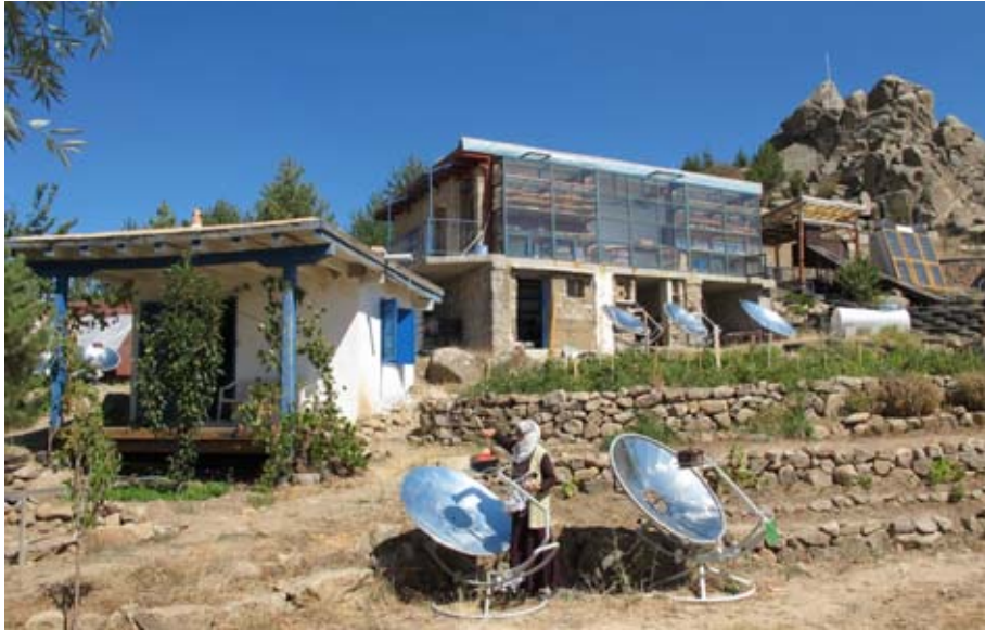
Figure 6. The Solar Building and solar cookers are part of the facilities provided by the Kerkenes Eco-Center. (10kecg0301)
