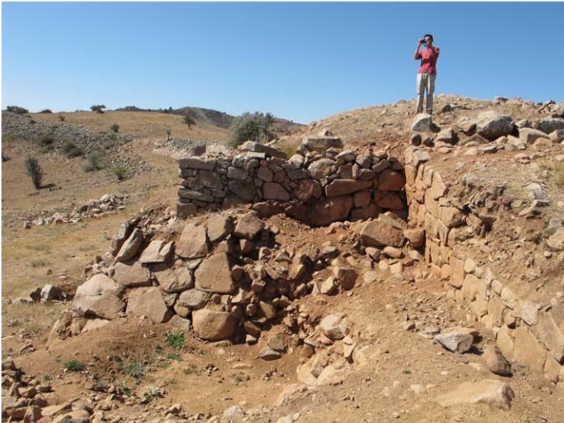
Figure 116. The East Tower, in September, before excavation of its northeast face. (10dpcg0206)
