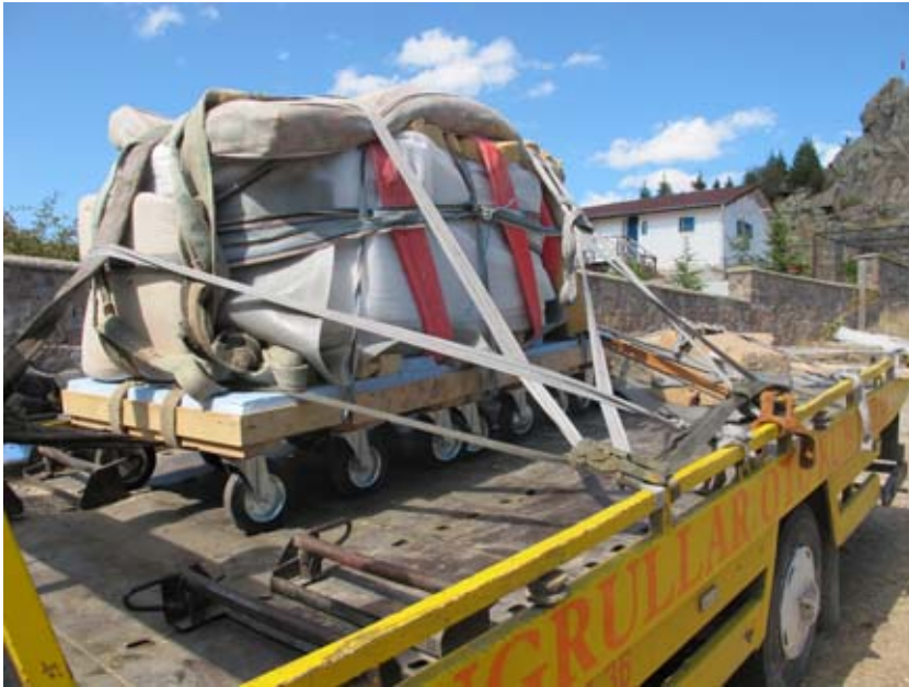
Figure 89. The plinth was wrapped up and moved on the heavy-duty trolley. (11dpcg3309)
