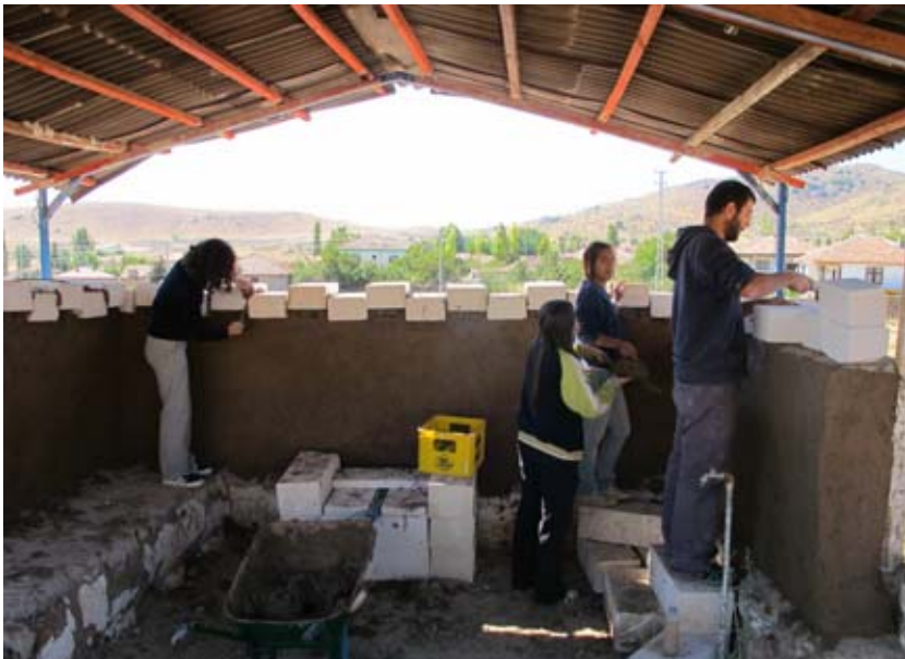
Figure 22. Architecture students combining traditional and modern materials in an experimental shelter. The Autoclave Aerated Concrete (AAC) blocks were donated by AKG Gazbeton. (11kecg1318)
