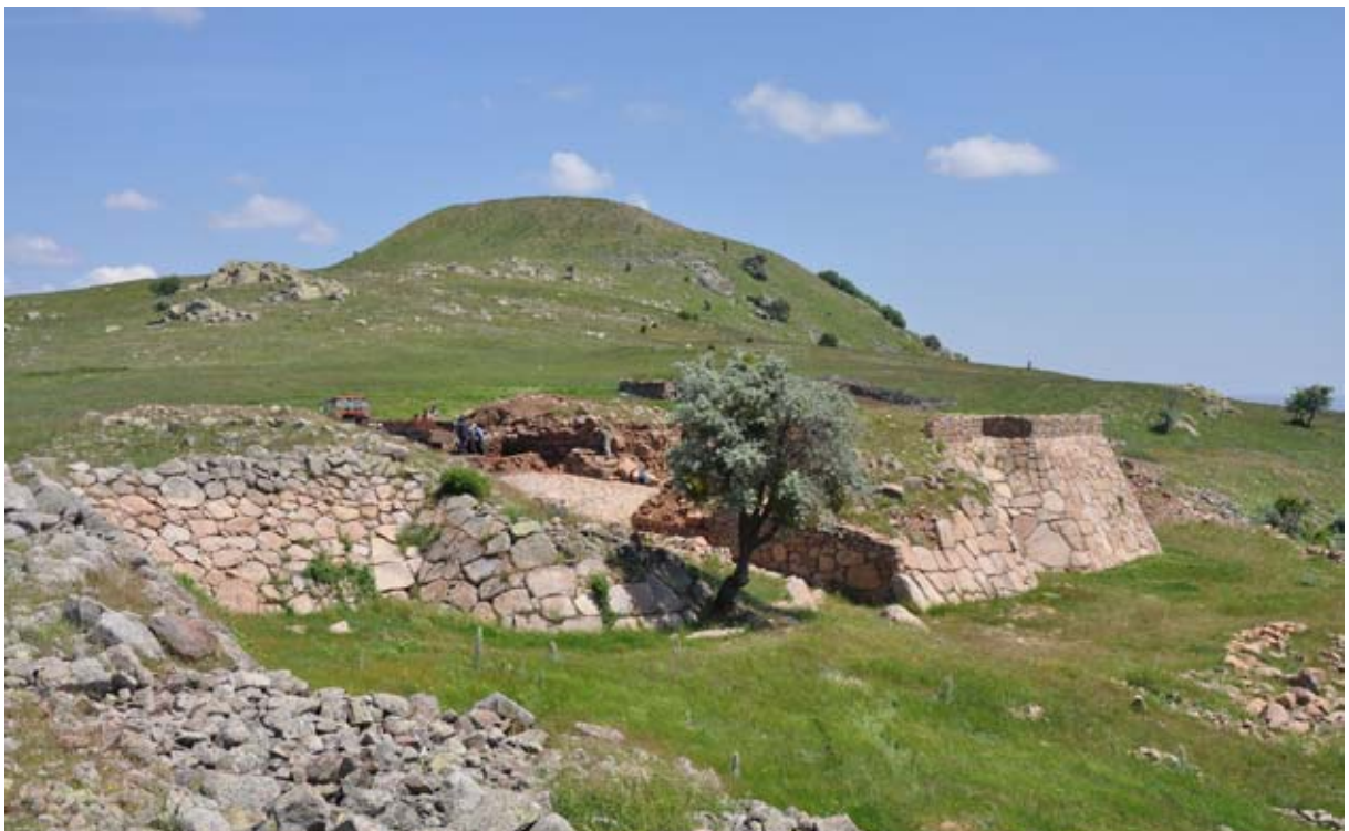
Figure 74. The Cappadocia Gate in June 2011. The glacis of the East Tower was restored in 2010 with funding from the US Ambassadors Fund for Cultural Preservation. (11dpnd0701)
