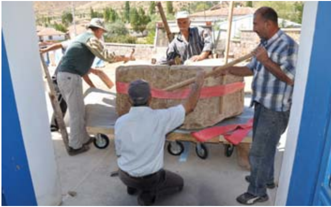
Figure 84. With the help of the stonemasons, the separate sections of the plinth core were brought together on the wheeled trolley. (11dpnd2008)
