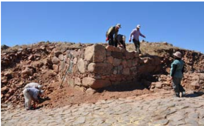
Figure 79. Repair of the West Tower in progress. (11dpnd2434)
