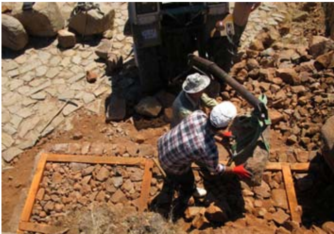
Figure 77. Large stones were lifted with the help of the tractor and its hydraulic lifting system. (11dpnd2434)
