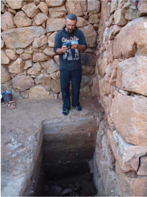
Figure 69. Trench supervisor Ferhat Can dug down to the base of the Middle Tower wall. (11dpkc2507)
