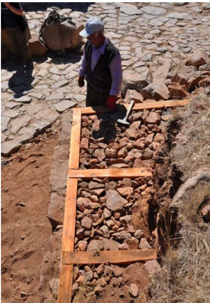
Figure 76. Stones were packed around the horizontal timbers. (11dpnd2356)
