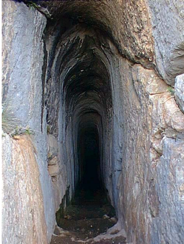
The rock-cut tunnel.
