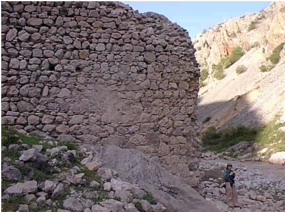
Detail of the wall with surviving timbers.
