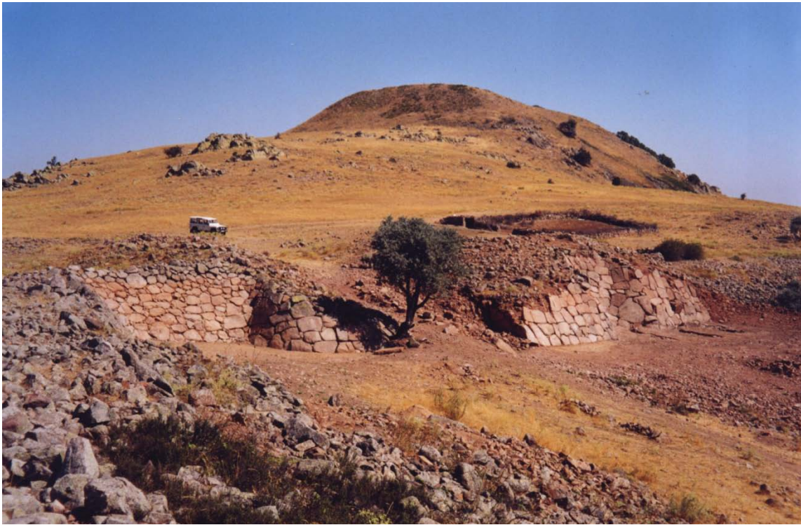
Figure 15: The steeply inclined stone glacis at the 'Cappadocia Gate' is fully preserved in the central niche of the double South-East Tower. The east wall of the gate passage is in shadow. The Kale forms a backdrop.
