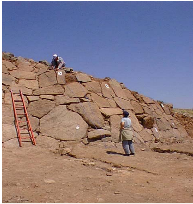
Figure 19: The stone glacis slopes at 45-60 and has rounded corners. Strings and control points mark out triangular planes on the glacis face to facilitate accurate measuring and rectification of photographs.
