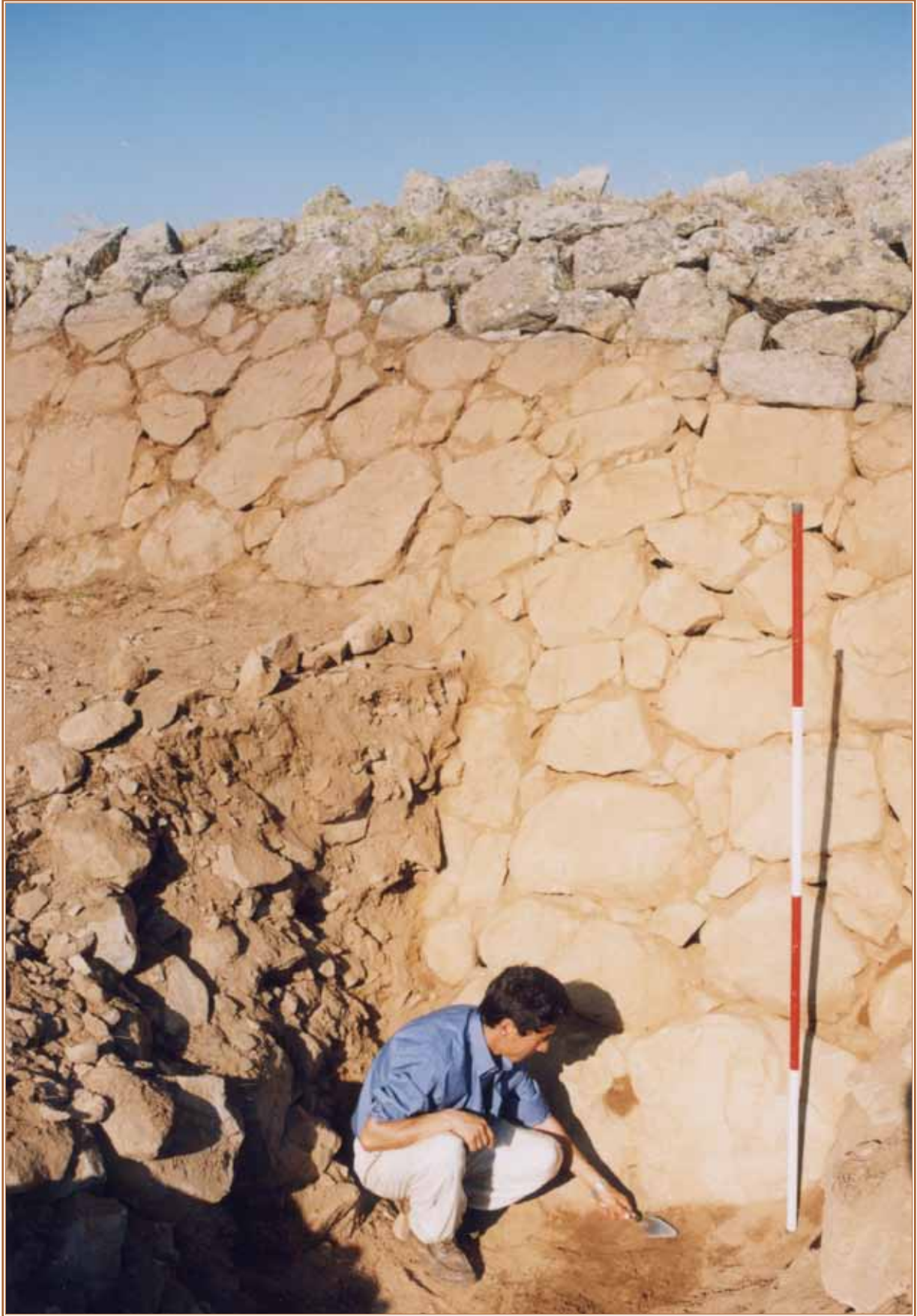
Figure 1: The sloping dry-stone glacis west of the Cappadocia Gate. Spaces between large cyclopean-like face stones are carefully chinked with smaller stones.
