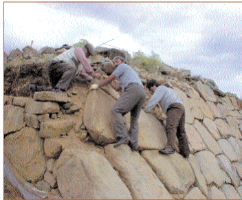
Figure 14: Repairing the glacis at the Cappadocia Gate.
