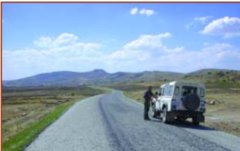
Figure 5. The new tarmac road winds all the way up to the site. Þekil 5. Dađ yamacýna uzanan yeni asfalt yol.
