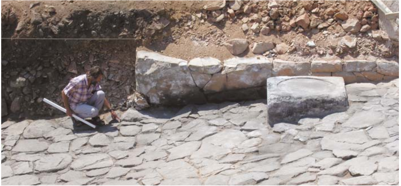
Figure 11. The east end of the South Tower and sandstone column base. Shattered stone blocks have been removed, for safety, revealing the loose rubble core of the tower.
