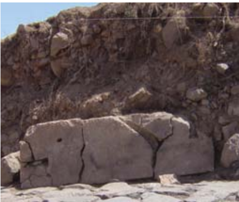
Figure 10. Large sandstone block, fallen from the front corner of the South Tower, with 3 clamp cuttings (at left, diagonal right of centre and at right).
